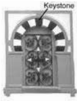
A keystone at the center of an arc above a doorway maintains its structure and support.
