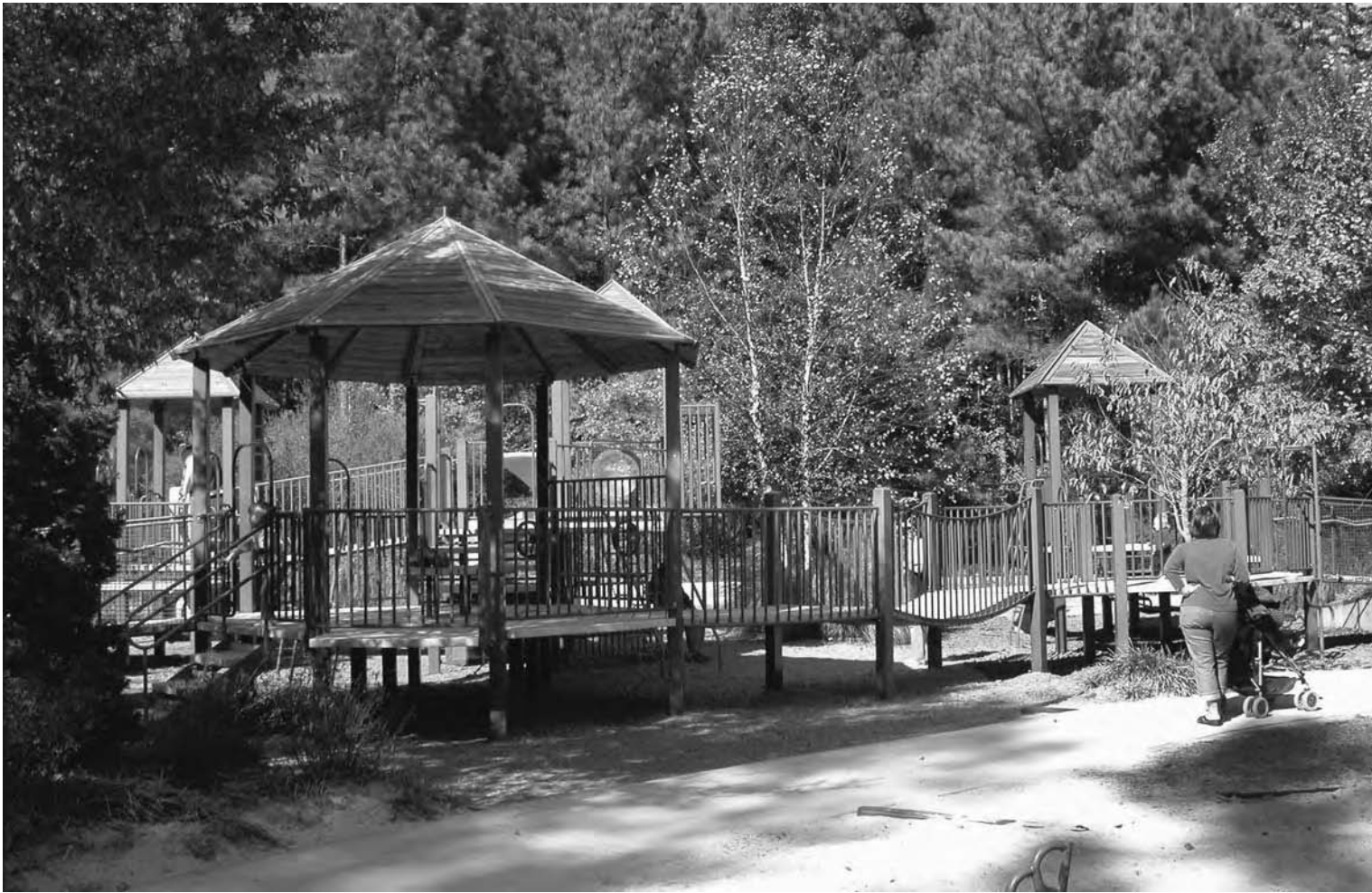
7.9 Zone 5: Horizontal composite structure – large swings, other equipment settings, sand play, accessible sand play, secondary path.
