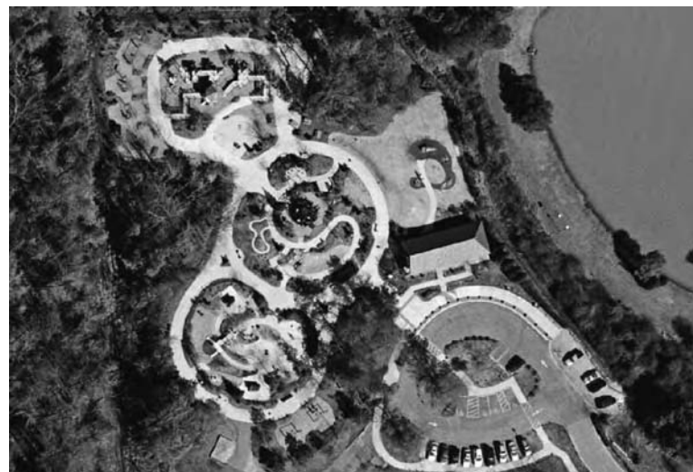
7.2 Aerial view of Kids Together Park, soon after construction.
