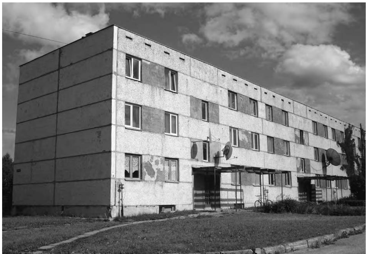
5.5 A Soviet-era block of flats in a village in Latvia, typical of the housing built during the collectivisation period.
