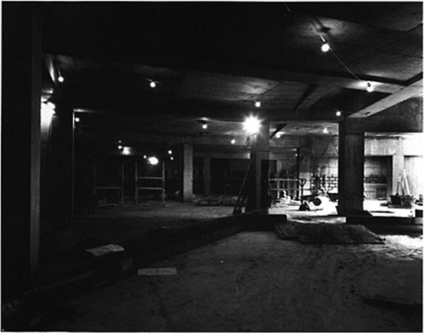
Figure 13.13 The Yorvik Viking Centre, York, under construction. (Source: York Archaeological Trust.)
