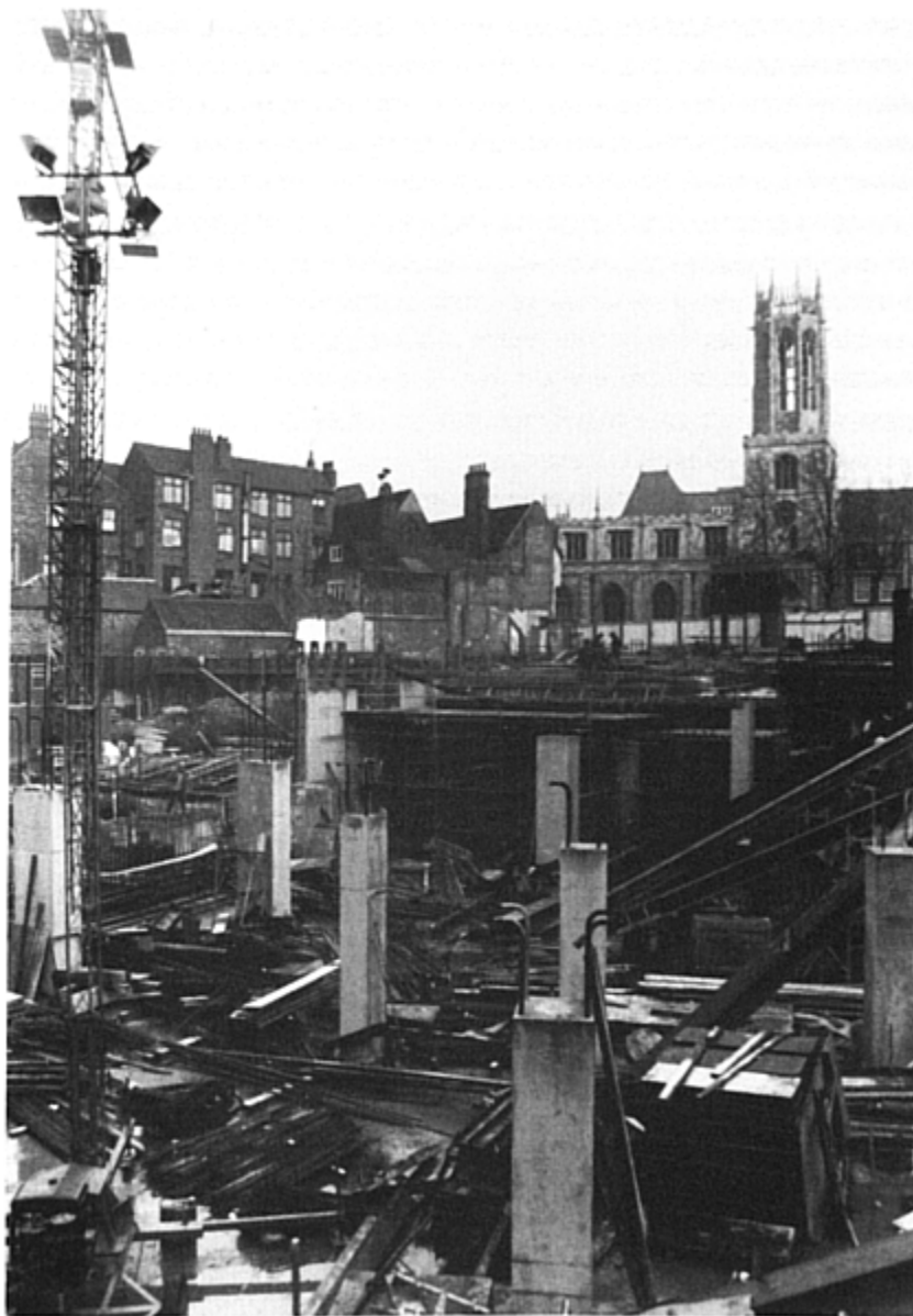
Figure 13.12 The Coppergate development, York, under construction. (Source: York Archaeological Trust.)
