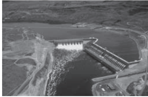
A run-of-the-river hydroelectric plant
