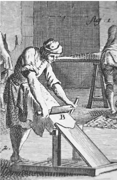
Figure 7.7 Shaving leather to uniform thickness.
