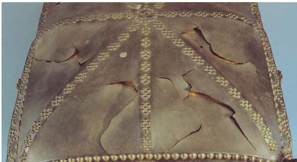
Figure 23.25 The roof, before treatment.
