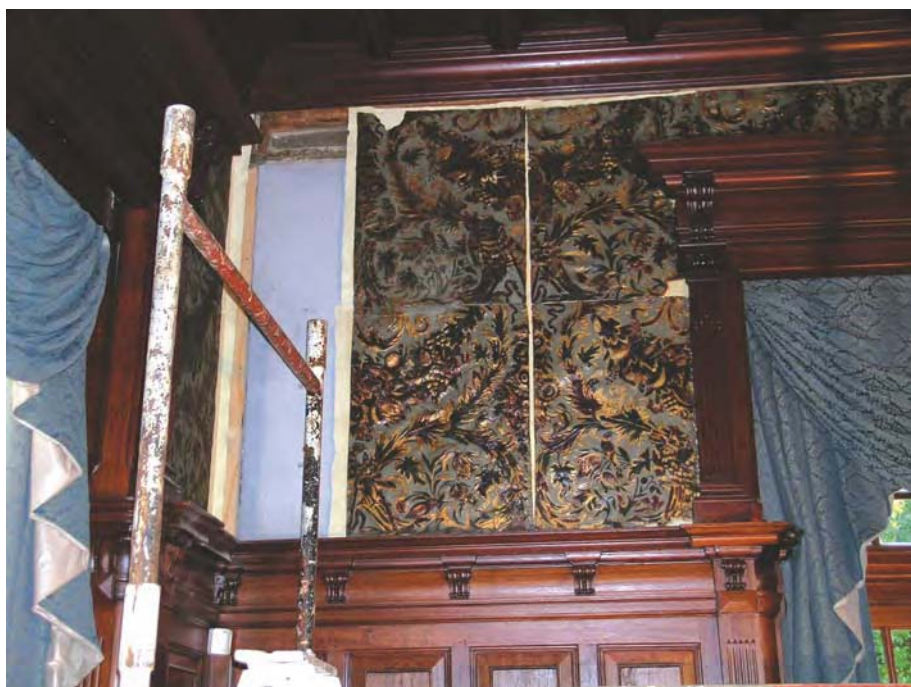
Figure 23.98 Some panels back on wall.
