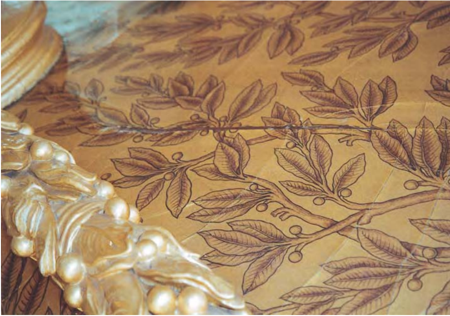
Figure 23.3 The finished repair. Inpainting still to be carried out.
