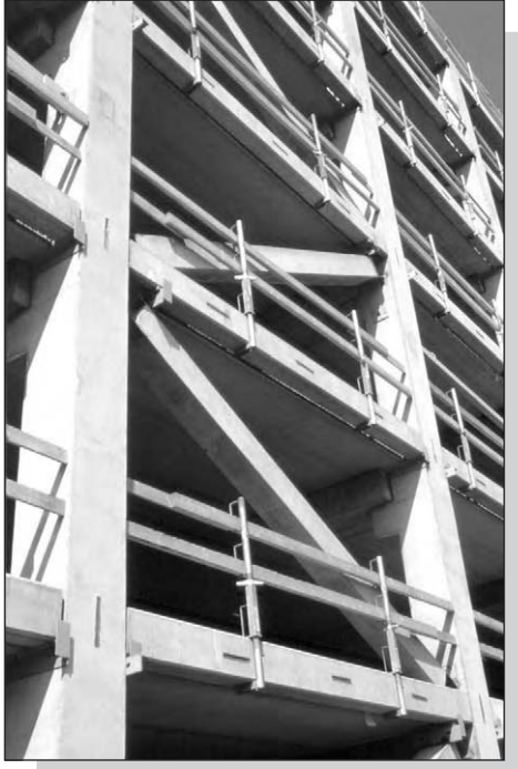
Figure 6.23: Concrete strut diagonal bracing.
