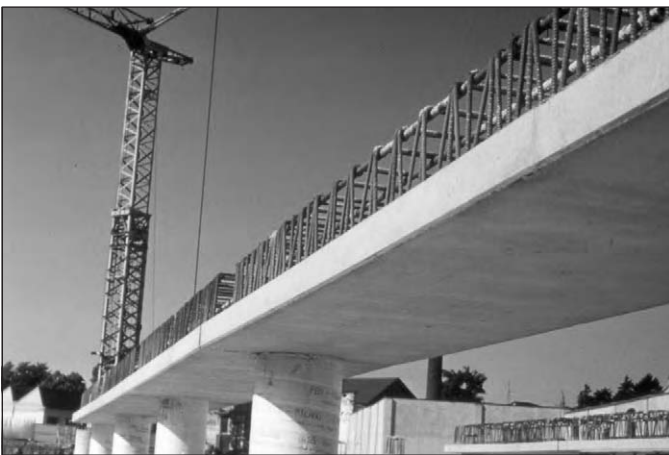
Figure 5.22: Precast concrete element with rebar girder awaiting composite action with the floor slab.
