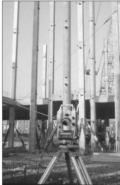
Figure 6.10: Stabilizing columns with compression props and guy ropes.
