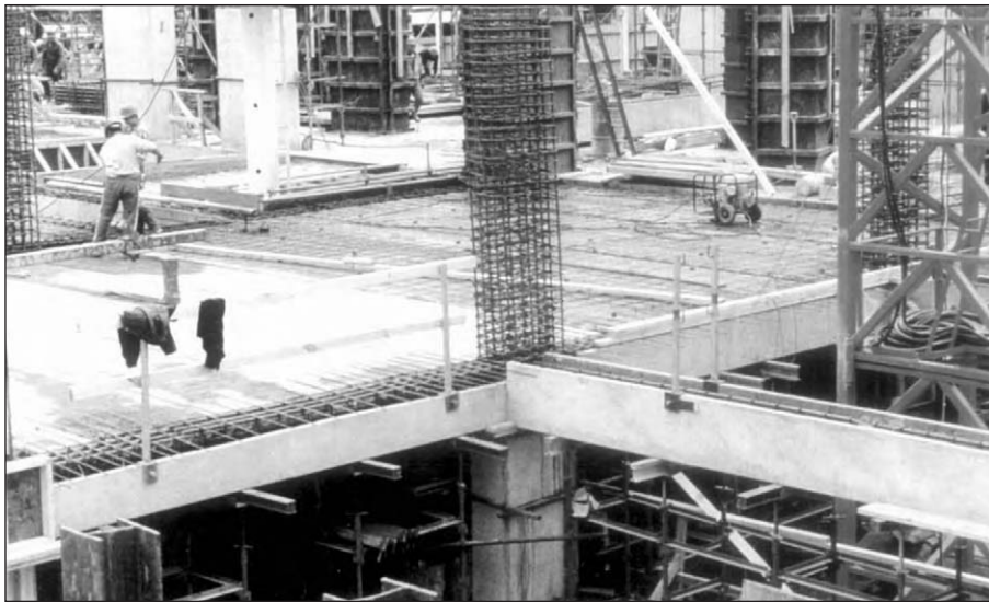
Figure 3.20: Precast U-beams awaiting cast in situ concrete filling.
