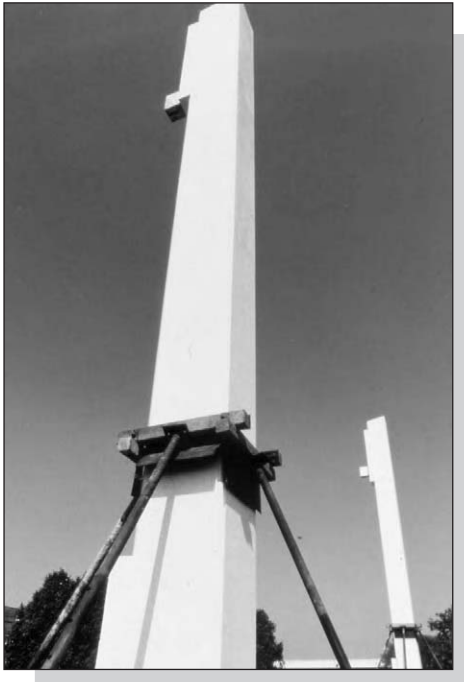
Figure 1.15: Polished columns resulting from the actions in Figure 1.14 (courtesy Trent Concrete, UK).
