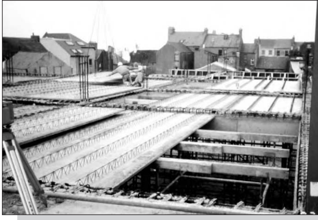
Figure 4.26: Propping of composite plank floor.
