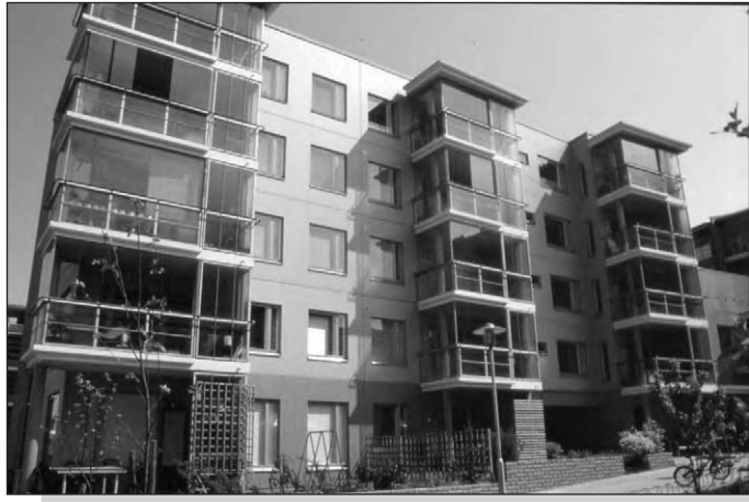
Figure 1.10: Precast concrete dwellings in a prefabricated concrete town.
