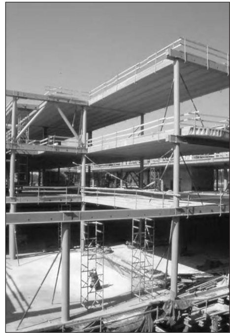
Figure 1.11: Mixed precast and structural steelwork construction.
