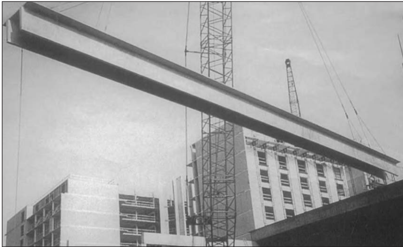
Figure 4.4: Double-tee floor slabs at a Missouri conference centre (courtesy PCI Journal, USA).
