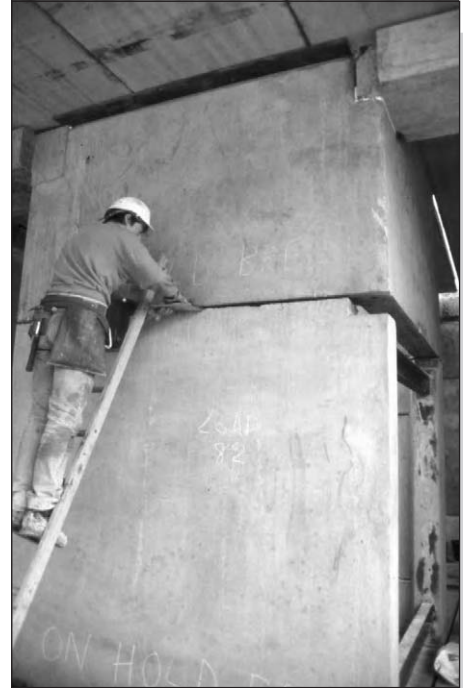
Figure 6.31: Dry packing between precast concrete walls.
