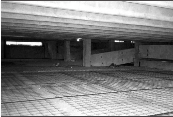
Figure 7.15: Laying a structural topping onto a precast double-tee floor.
