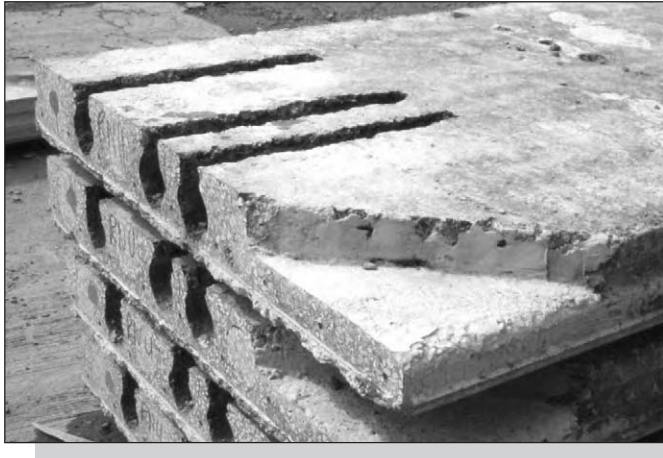
Figure 10.6: Corner recess in hollow core slabs to permit the correct placement of ties at corners.
