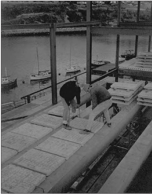
Figure 4.6: Composite beam and plank floor under construction.
