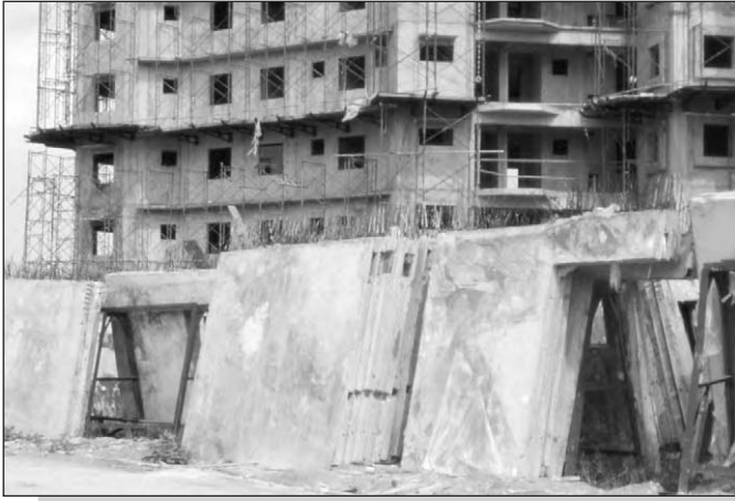
Figure 1.2: Site cast precast concrete.
