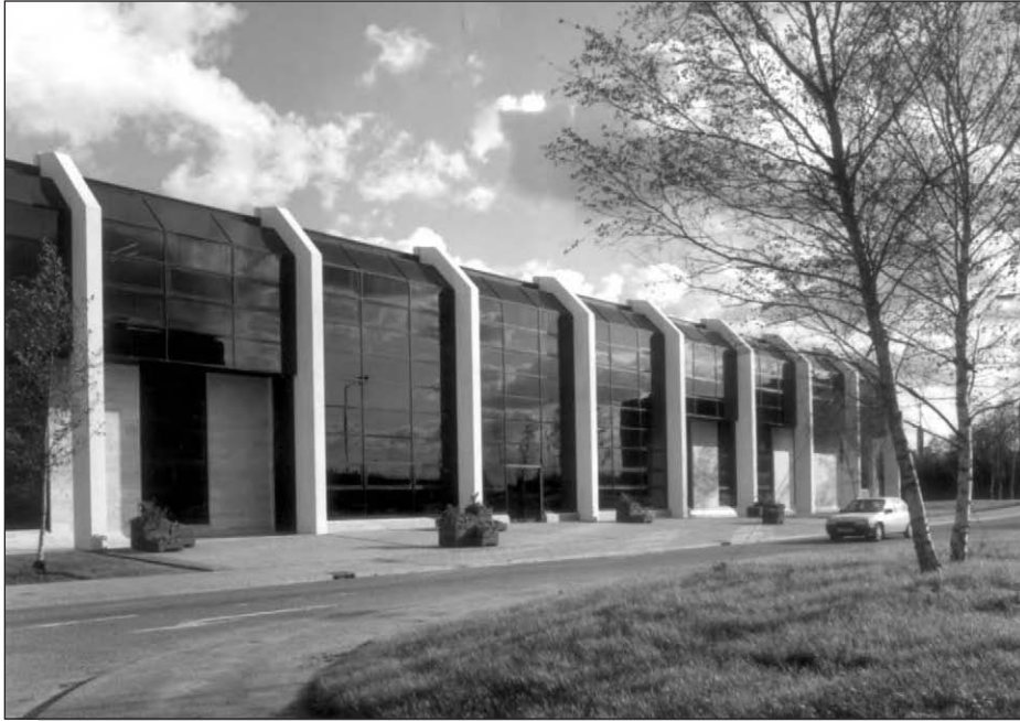
Figure 6.2: White concrete columns at Sunbury Business Centre, UK (courtesy British Cement Association, UK).
