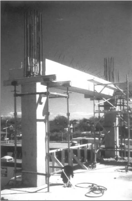
Figure 8.31: Moment continuity reinforcement placed in precast U-beams.
