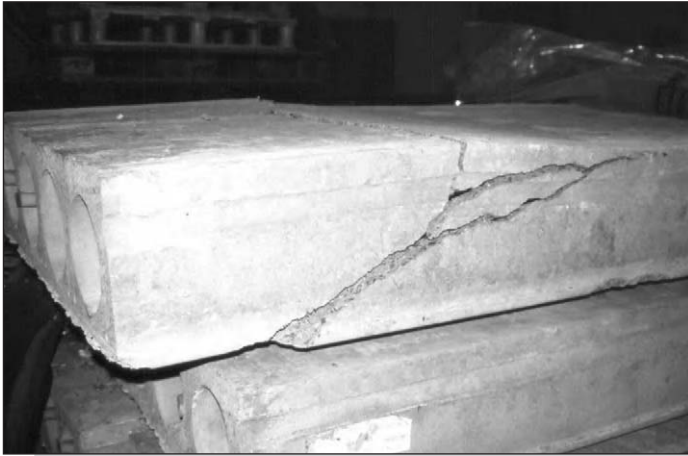
Figure 4.19: Shear failure in prestressed hollow core slab.
