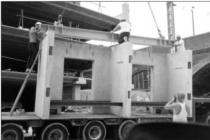
Figure 6.22: Storey height precast lift shaft units.
