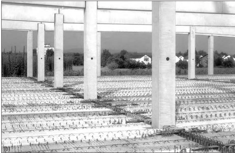
Figure 4.8b: Practical layout of composite plank flooring (courtesy Pfeifer Seil und Hebetchnik, Memmingen, Germany).
