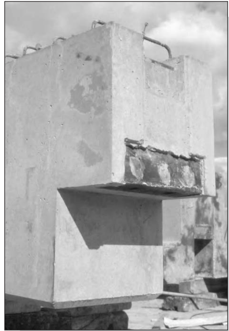
Figure 9.16: Recessed beam end connection to rectangular beam.
