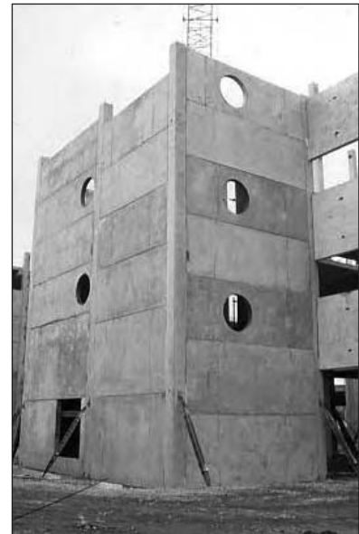
Figure 6.19: Precast concrete infill walls.
