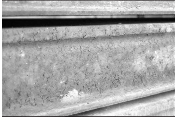
Figure 7.11: Edge profile of slip-formed hollow core slab.
