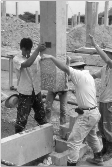
Figure 9.4: Column-to-foundation connection using grouted pocket.
