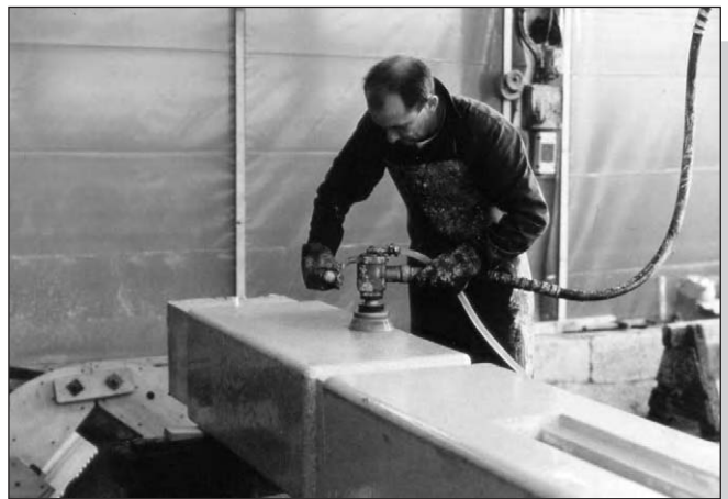
Figure 1.14: Polishing concrete to create pseudo marble finishes (courtesy Trent Concrete, UK).
