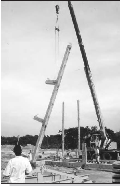
Figure 6.9: Pitching asymmetrical columns.
