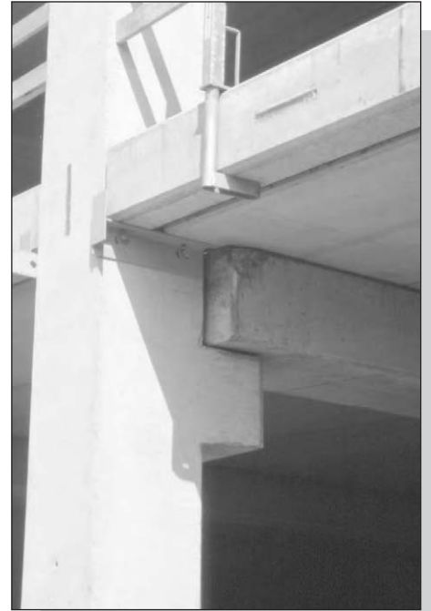
Figure 1.3: Simple bearing nib.
