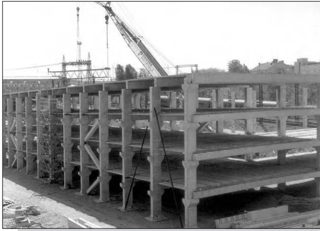
Figure 9.33: Corbel connections at Hartwell Arena car park, Finland (courtesy Betoni).
