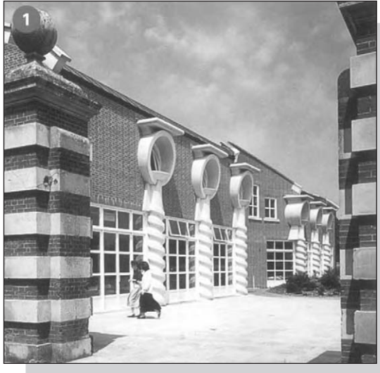
Figure 1.16: Precast spirals adorn Braynston School, UK (courtesy Techcrete Ltd, Ireland and UK).
