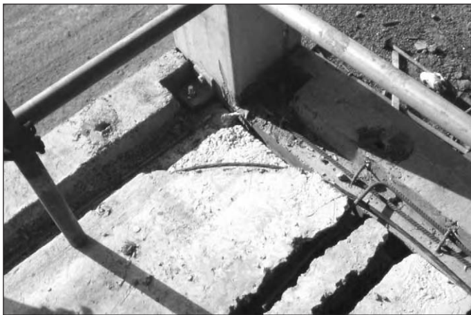
Figure 10.5: Continuity of beam ties at corner columns.
