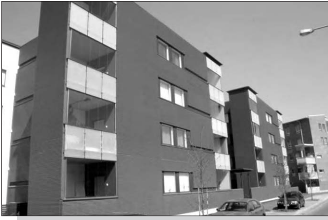
Figure 3.4: Exterior facade to wall frame.
