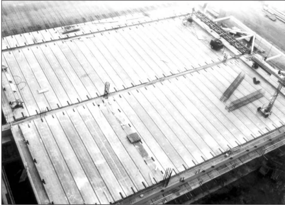
Figure 4.1: Hollow core floor slabs (courtesy Bevlon, Association of Manufacturers of Prefabricated Concrete Floor Elements, Woerden, Netherlands).
