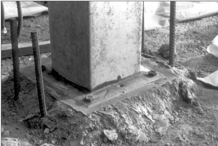
Figure 9.3: Column-to-foundation connection using extended steel base plate.
