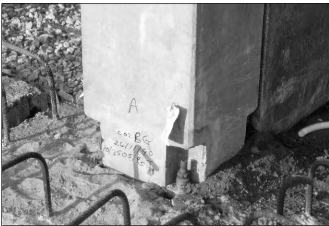
Figure 9.43: Column-to-foundation connection using flush steel base plate.
