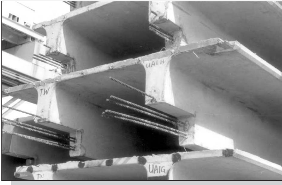
Figure 4.5: Double-tee end profile – the half joint is to raise the bearing level and reduce structural depth.
