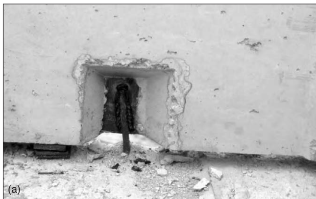
Figure 8.23a: Welded connection between rebar and plate.
