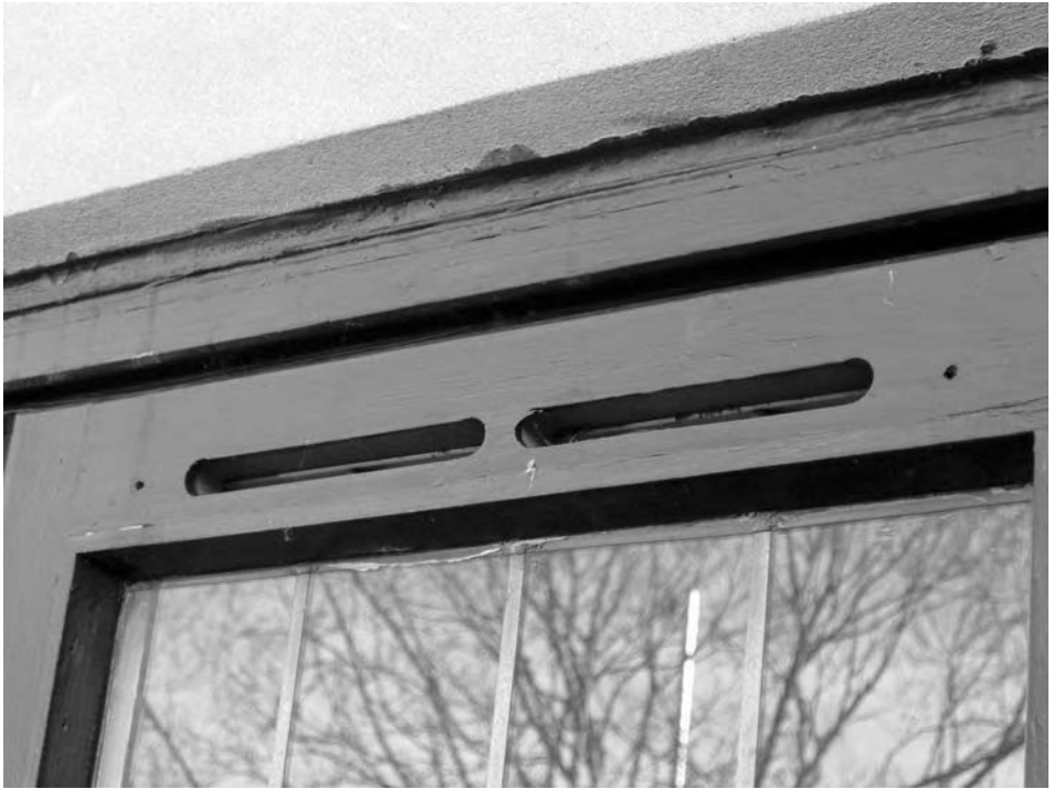
Figure 7.3 Routed slit in window frame for trickle ventilation
