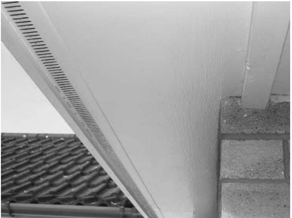
Figure 7.8 Trickle ventilator continuous strip
