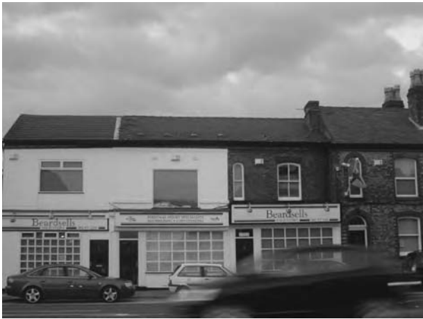
Figure 5.5 Tile ventilator terminals on roof
