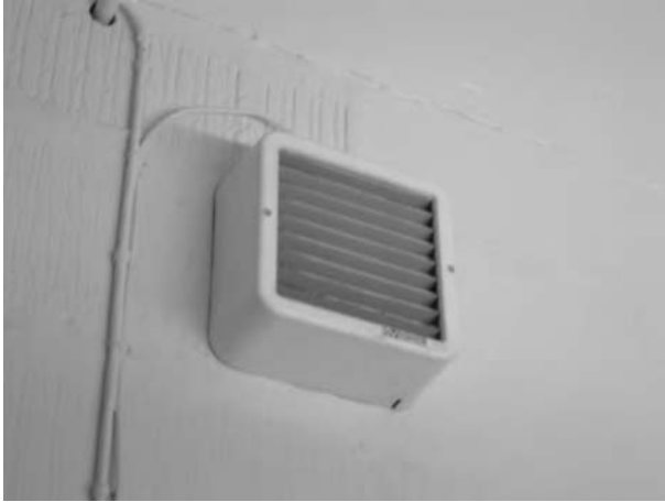
Figure 5.8 Typical domestic extract fan
