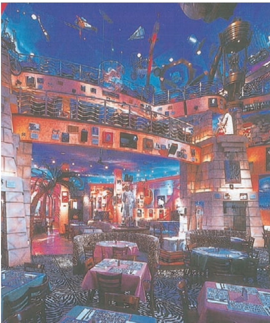
Plate 26 Planet Hollywood in Walt Disney World Orlando, USA, 1994, architect and interior designer: Rockwell Group). A building with entertainment restaurants, it is a translucent blue globe over 30 m high, at night covered with shimmering coloured lights. © {ai; Warchol.
