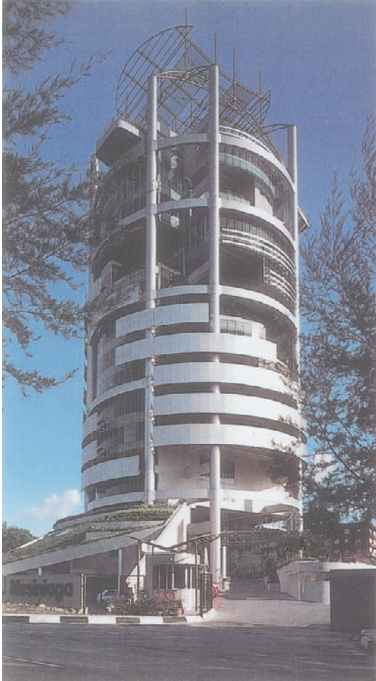
Plate 16 Menara Mesianaga, Kuala Lumpur, Malaysia, 1992. Fourteen-storey building, post-modern in a developing country; side core building, metallic external skin, 'sky-courts'. © Harrison et al.: Intelligent Buildings in South East Asia , E & FN Spon.
