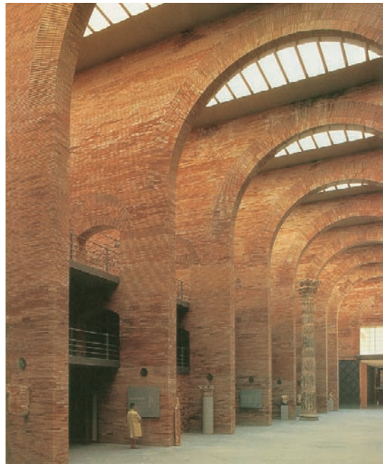
Plate 18 National Museum of Roman Art, Merida, Spain, 1980–85, architect: José Rafael Moneo. Modern architecture with the use of traditional materials: (Roman style) brick masonry bearing walls, filled with concrete. © The Pritzker Architecture Prize .
