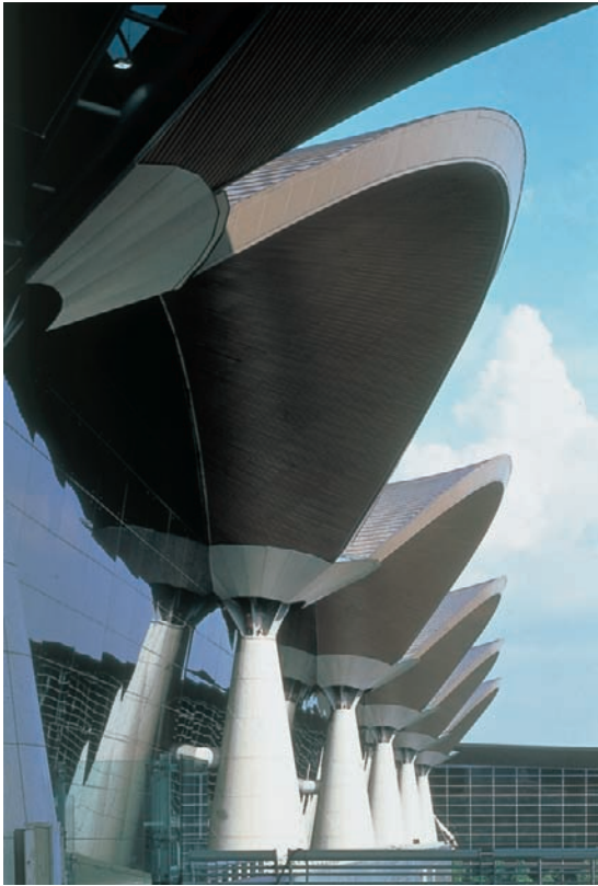
Plate 22 Kuala Lumpur International Airport, Malaysia, architect: Kisho Kurokawa.
