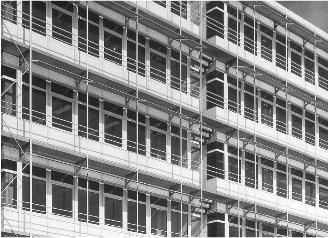
Figure 4.5 Town Hall, Emsdetten, Germany, horizontal shading elements. © Courtesy of Shüco, Bielefeld.
