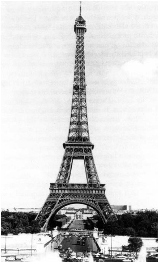
Figure 1.1 The Eiffel Tower, Paris, France, 1887–89, structural design: Gustave Eiffel, 300 m high. One of the first spectacular results of technical progress in construction. © Sebestyen: Construction: Craft to Industry , E & FN Spon.
