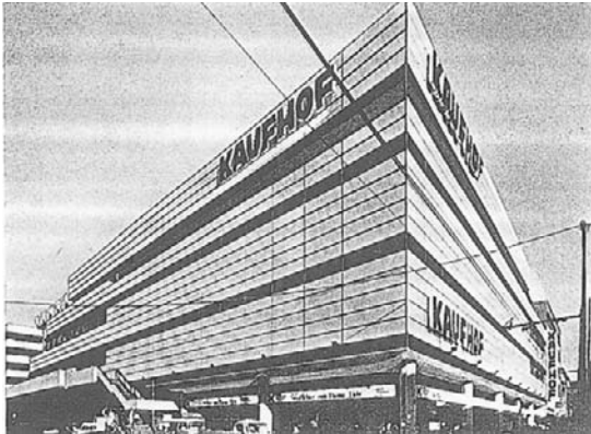
Figure 3.5 Façade system (two variants) with aluminium frame sections, fixed insulating glazing and plastic spacers (Mesconal, Germany). © Sebestyén: Lightweight Building Construction , Akadémiai Kiadó.
