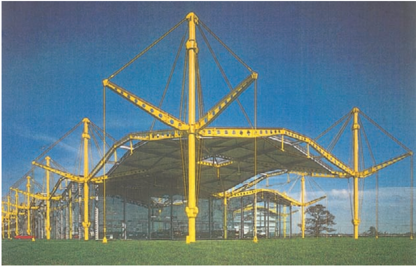
Plate 10 Renault UK Distribution Centre, storage depot, Westlea Down, Swindon, Wiltshire, UK, 1982–83, architect: Foster Associates, structural engineer: Ove Arup and Partners. Masted building, suspended roof, coloured appearance.
