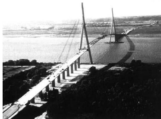
Figure 1.5 Cable-styled bridge, Pont de Normandie, France; main span: 856 m. Source: Freyssinet Photo Service.
