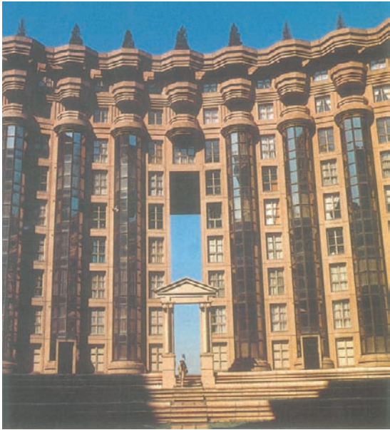
Plate 4 Les Espaces d'Abraxas, Marne-la-Vallée, France, 1979-83, architect: Ricardo Bofill. Neo-historic architecture designed with pre-cast concrete components.
