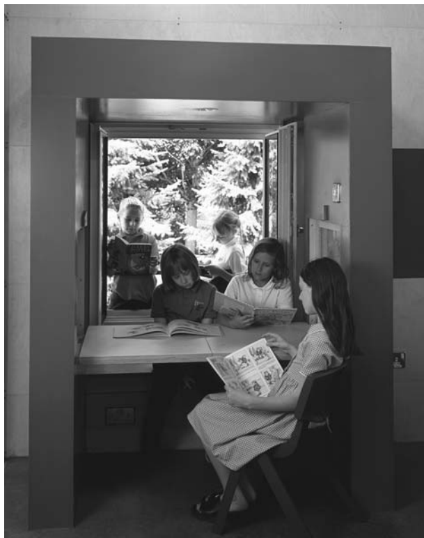
Figure 6.4 Box bay open makes a connection between the inside and outside spaces.
