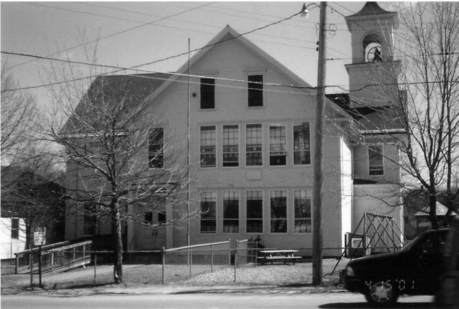
Figure 4.1 Elm Street School, Camden, Maine, 1869. (Photo: Eleanor Nicholson.)
