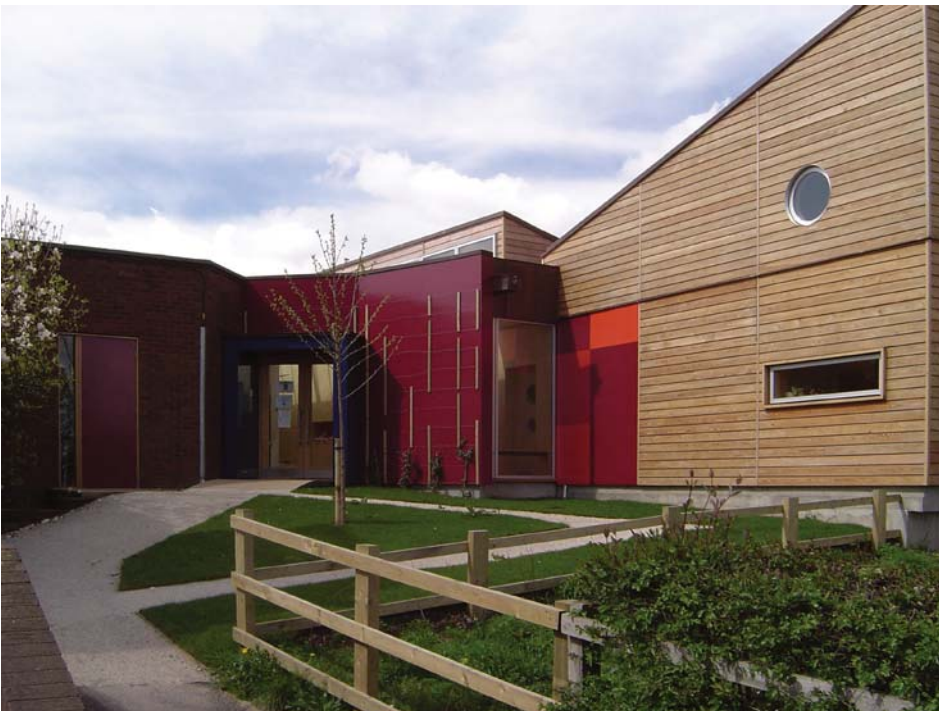
Plate 8 Ballifield Community Primary School, Sheffield: new entrance and classroom. (Architect: Prue Chiles.)
