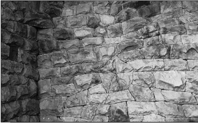
Figure 13.10: Dry-stone walling of specially cut stone.
