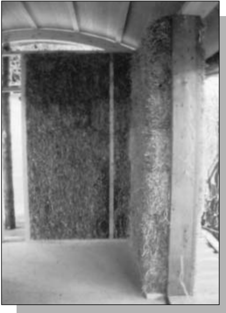
Figure 14.17: Straw bale building. Source: Howard Liddell
