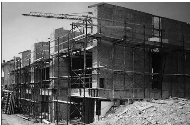
Figure 14.14: Dwellings built with woodwool blocks under construction in Italy.
