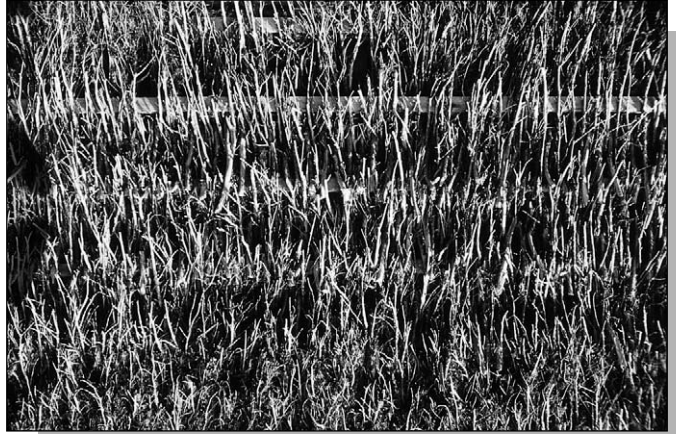
Figure 15.23: Detail of bracken cladding. Source: Dag Roalkvam
