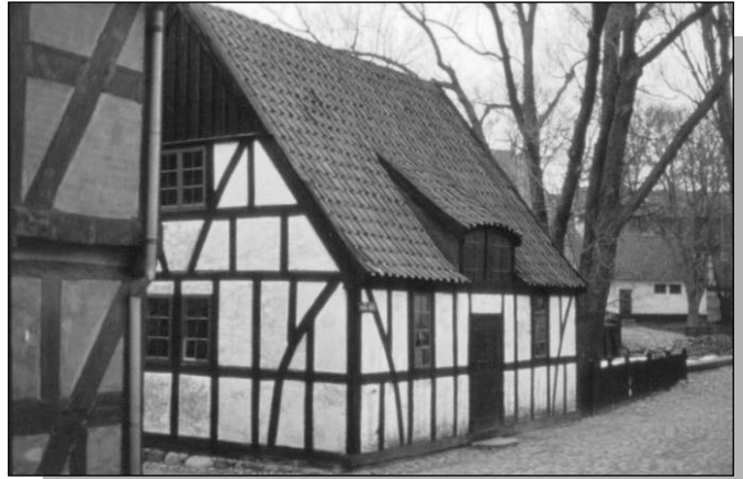
Figure 13.41: Traditional way of filling spaces with brick in a timber framed building in Denmark.
