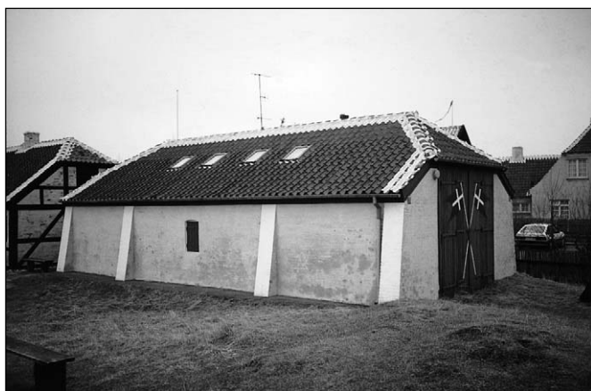
Figure 13.15: A small Danish building entirely constructed in fired clay without using reinforcement.
