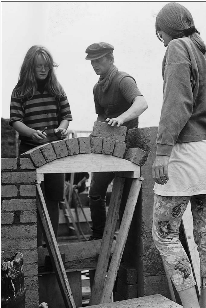
Figure 13.25: Building with earth blocks. Source: Gaia Lista 1991
