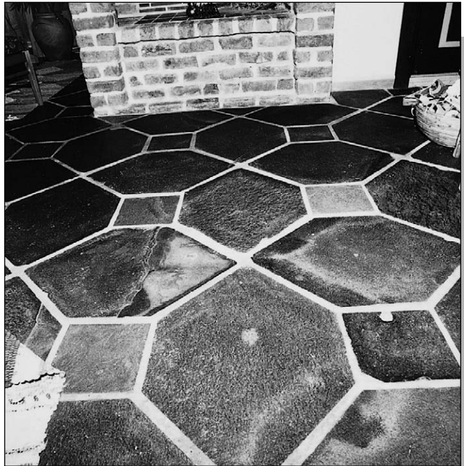
Figure 15.4: Floor covering of slate, mixed with old roof slates. Source: Gaia Lista, 1990
