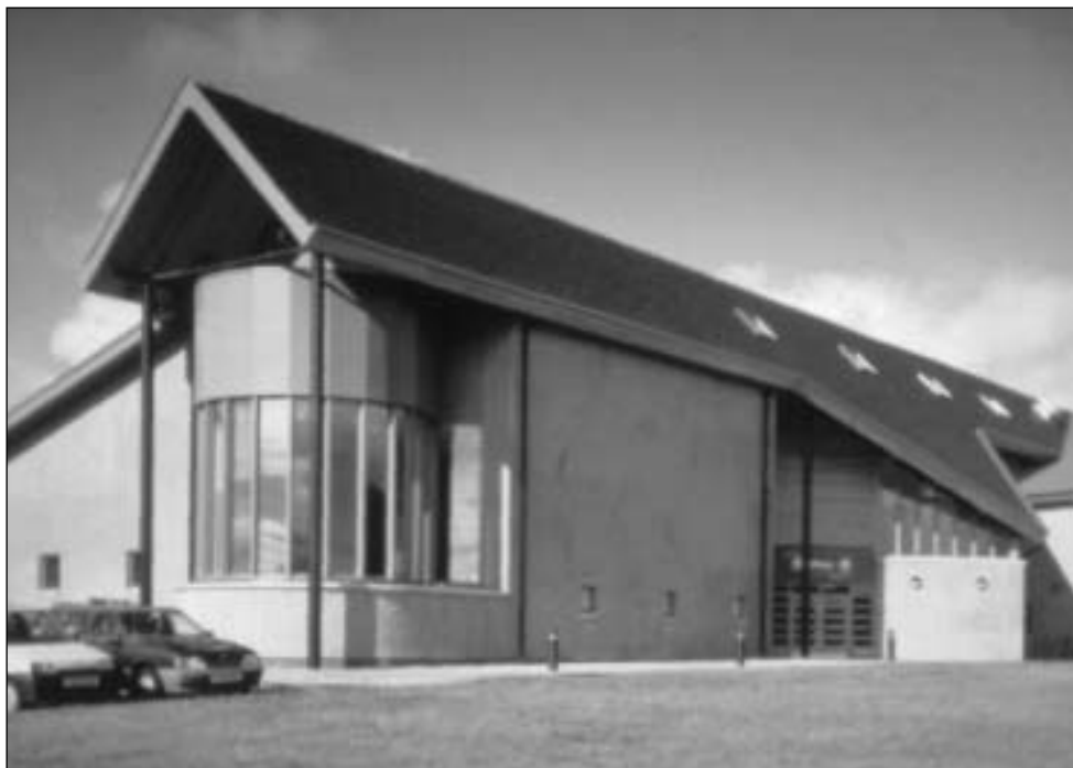
Figure 14.2: The McLaren Leisure Centre, Callander: a healthy building materials specification, with dynamic insulation in the ceiling. Source: Howard Liddell
