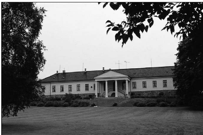
Figure 13.26: The manor house of Skinnarebøl in south east Norway from the early 19th century is built in the wet-formed wall technique.
