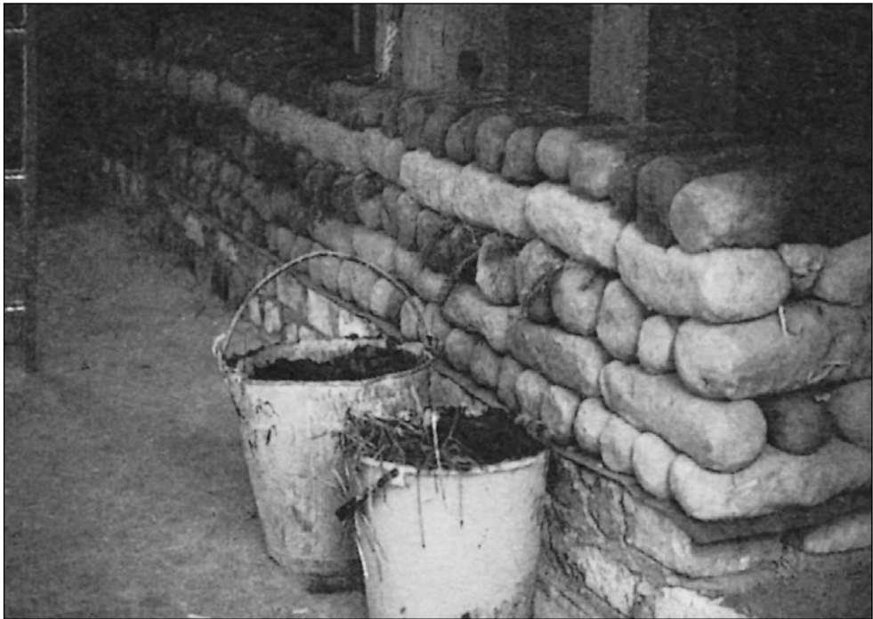
Figure 13.27: The earth loaf technique.
