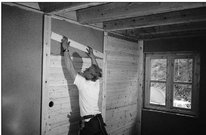
Figure 15.21: The construction of demountable internal panelling.
