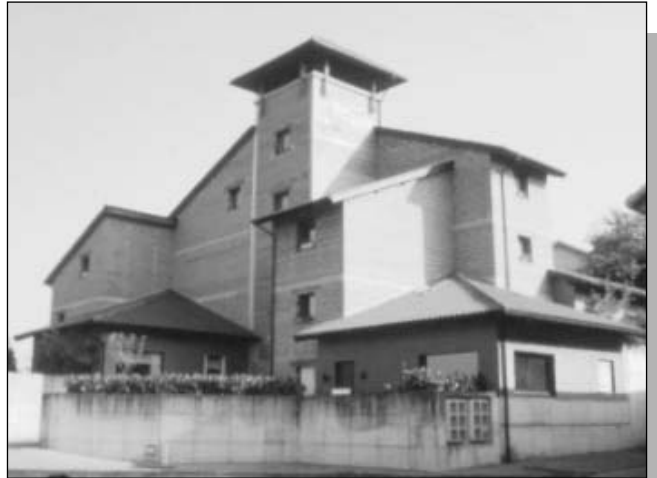
Figure 8.4: Earth building at Ile d'Abeau in France by architects F. Jourda and G. Perraudin.
