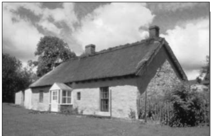
Figure 13.18: Recently renovated 200-year-old earth building in pisé construction in Perthshire. Source: Howard Liddell
