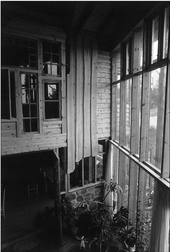
Figure 16.2: Use of recycled windows in a house, between the living room and the garden. Source: Gaia Lista 1986
