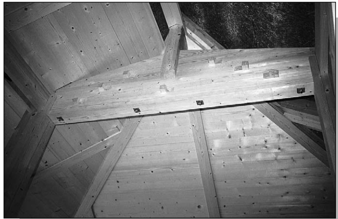
Figure 13.29: A roof joint bolted together, not glued, stiffened by dowels. Source: Gaia Lista, 1987
