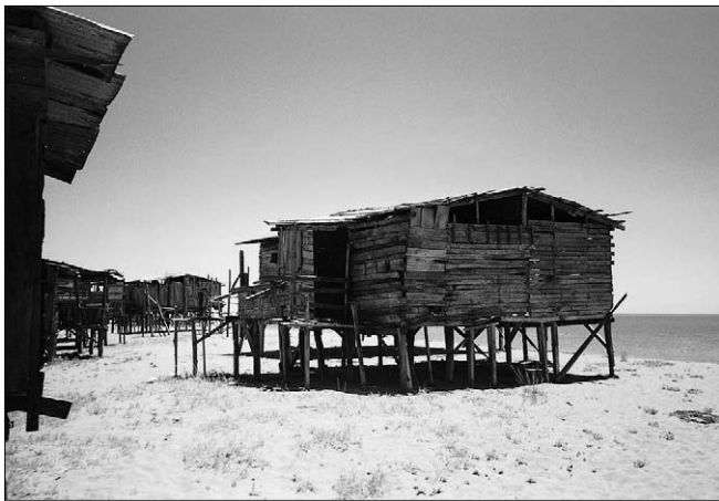
Figure 1.2: A traditional summer village on the south coast of Turkey. The huts are made of driftwood, packing cases, packaging and other available free material, and are used as summerhouses by the local population.
