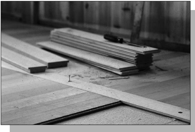
Figure 15.24: Batten flooring under construction.
