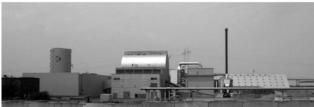
Cogeneration on the larger scale is well established – this Danish plant burns more than 60,000 t of straw a year, and produces 8.3MW of electricity and 20.8MW of heat
