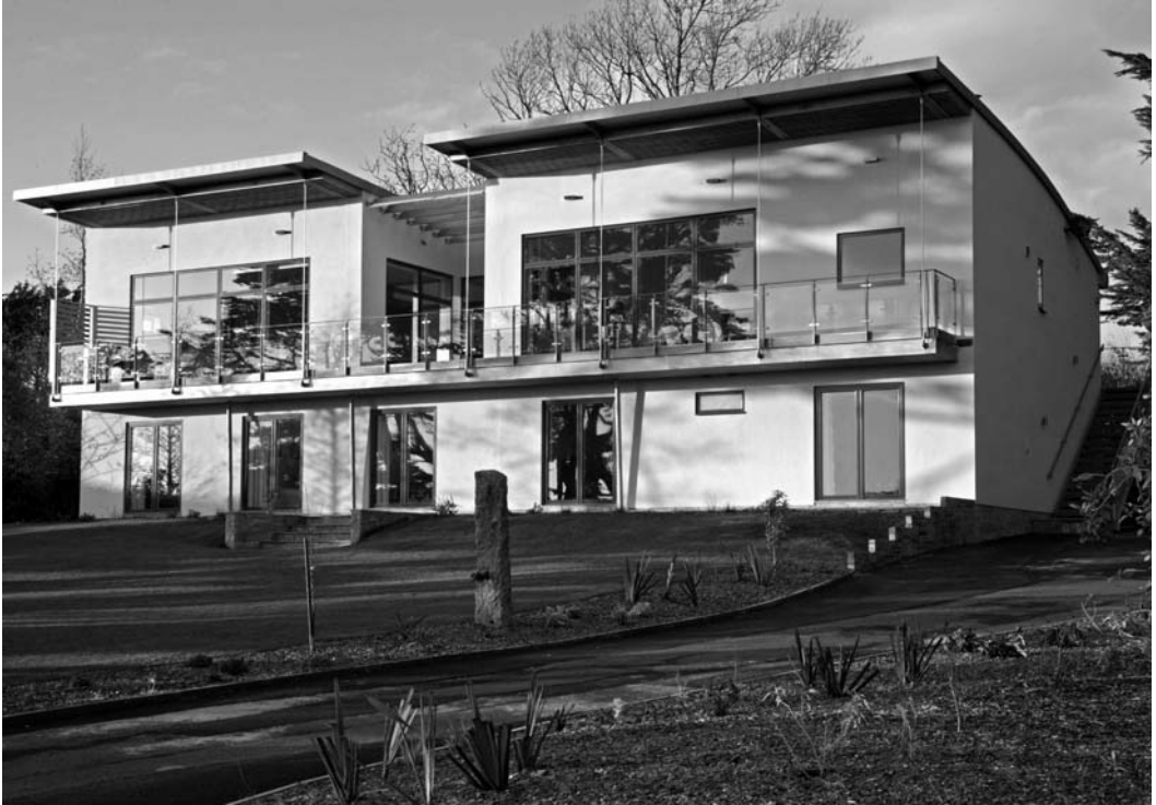
An 'upside-down' layout and high thermal mass shape the architecture of this holiday home (Reproduced with permission from Clive Boursnell)
