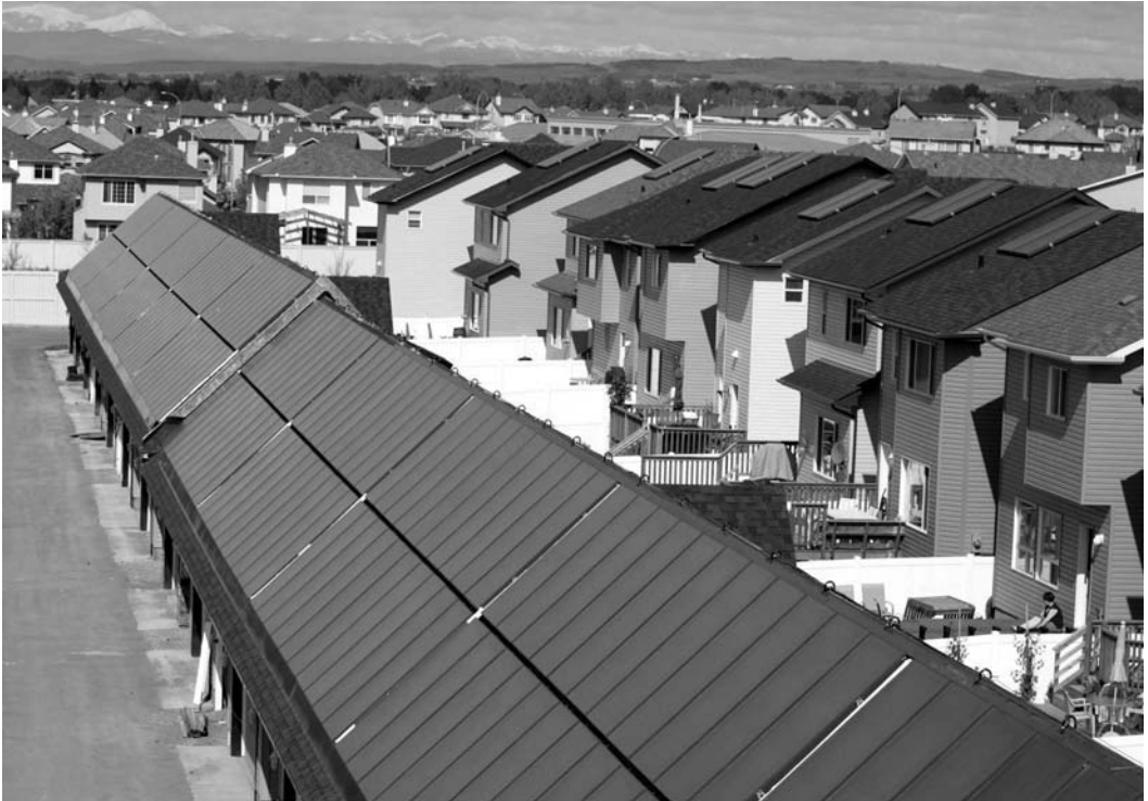
Solar energy is captured by flat plate collectors on garage roofs (Photo provided courtesy of Natural Resources Canada)
