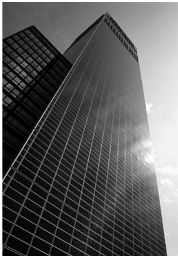
Manchester's CIS tower shows what PV can do in the right context (Reproduced with permission from Solarcentury.com)
