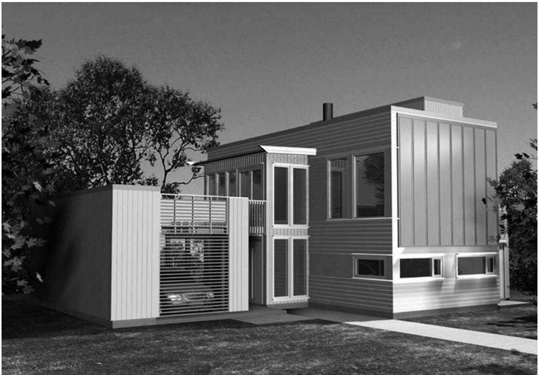
Conventional flat plate collectors can also be used on façades (Reproduced courtesy of Solarnor)
