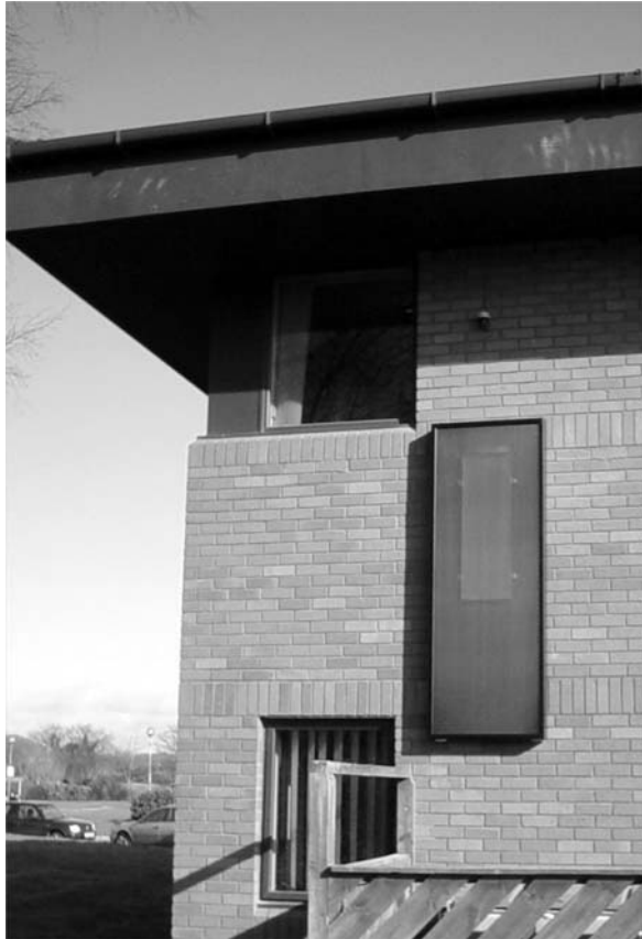
In higher latitudes TAPs are best mounted on façades (Reproduced with permission from SolarVenti)
