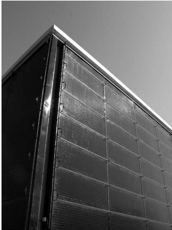
Façade cladding may be replaced by unglazed stainless steel or polymeric collectors in higher latitudes (Reproduced with permission from Energy Solaire)
