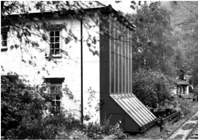
This Welsh house features both passive solar water heating and a Trombe wall (Reproduced with permission from Martin J. Pasqualetti)
