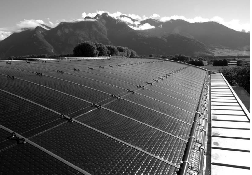
Unglazed stainless steel flat plate collectors can be curved for architectural effect (Reproduced with permission from Energy Solaire)
