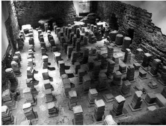
Roman underfloor heating was more sophisticated than the Korean equivalent shown below (Reproduced with permission from Akajune)
