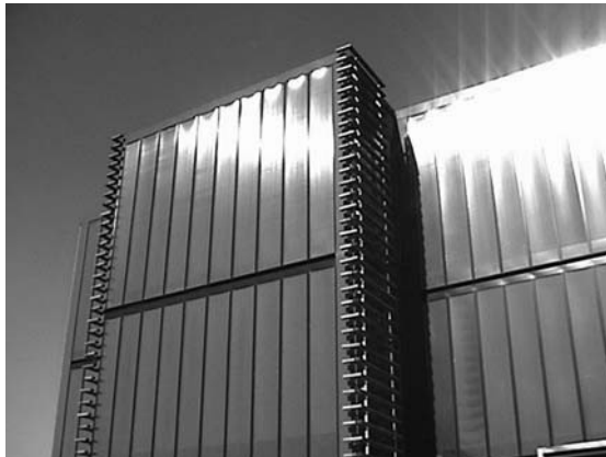
Façade-integrated collectors could be the best choice for solar water heating on tall buildings (Reproduced courtesy of Solarnor)
