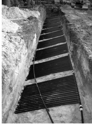
Horizontal 'Compact Collectors' from ICE Energy (Reproduced with permission from ICE Energy Heat Pumps)
