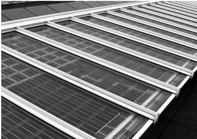
‘Translucent’ solar PV glazing continues to improve (above and below) (Reproduced with permission from Solarcentury.com)
