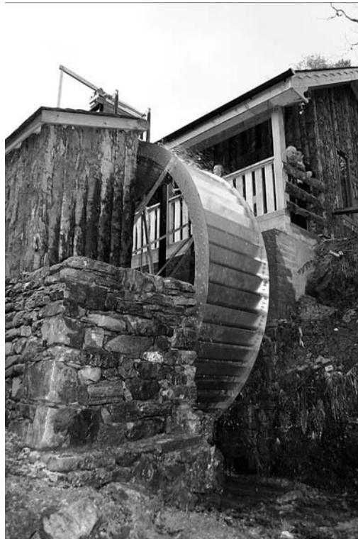
The Stornoway Waterwheel revives a 19th Century mill site (Reproduced with permission from Tony Robson Consultant)
