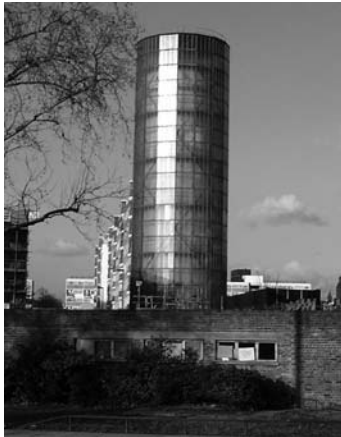
Hot water from London's Battersea Power Station was stored in this 'accumulator' – a large thermal store – on the other side of the Thames and used to heat houses in Pimlico (Reproduced with permission from Fin Fahey)
