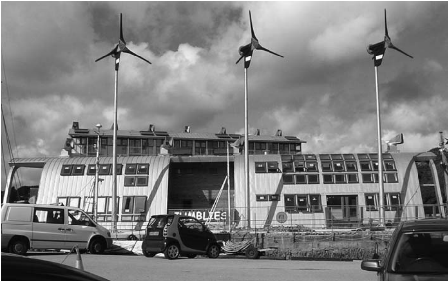
Mast mounting away from the building is usually a better solution than HAWTs on rooftops (Reproduced with permission from Proven Energy)
