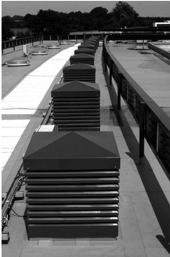
Modern multi-directional windcatchers are a well-developed option (Reproduced with permission from Monodraught)
