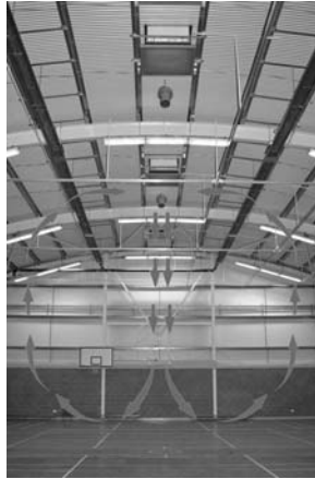
Monodraught's Heat Harvester recirculates warm air from under the roof (Reproduced with permission from Monodraught)
