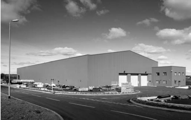
Buildings with façades made up of transpired air collectors look little different to conventional structures (Reproduced with permission from CA Group)
