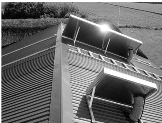
Thermosyphoning air panels offer a space heating solution for light industrial buildings (Reproduced with permission from SolarVenti)
