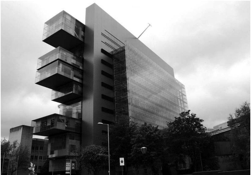
Cantilevered courtrooms are a distinctive feature of the Manchester Civil Justice Centre (Reproduced with permission from Mott MacDonald)
