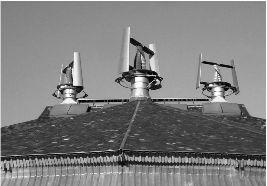
VAWTEX wind-powered extraction units (Reproduced with permission from Arup – Mike Rainbow)
