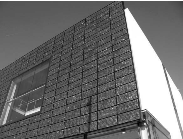
Solar cladding replaces more conventional alternatives (Reproduced with permission from Solarcentury.com)
