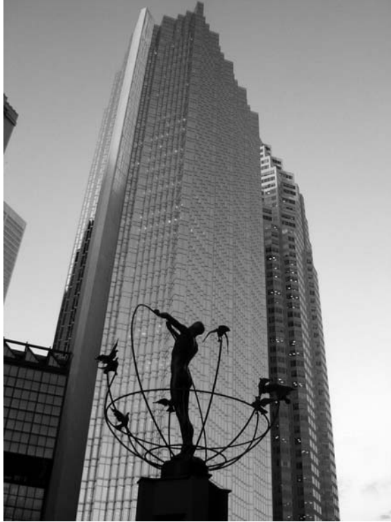
Once famous for the energy saving gold coating to its glazing – more than $1 million worth of gold was used – Toronto's Royal Bank Plaza is now cooled via the waters of Lake Ontario
