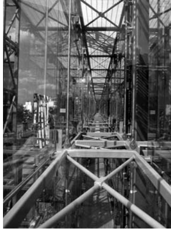
Passive cooling techniques can be incorporated into high technology buildings (Reproduced with permission from Mott Macdonald)
