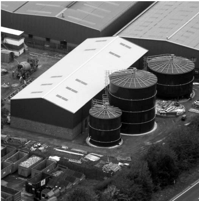
This anaerobic digestion unit in Shropshire, England, produces more than 1,600 MWh annually from 5,000 t of food waste and grass cuttings (Reproduced with permission from Greenfinch Ltd)
