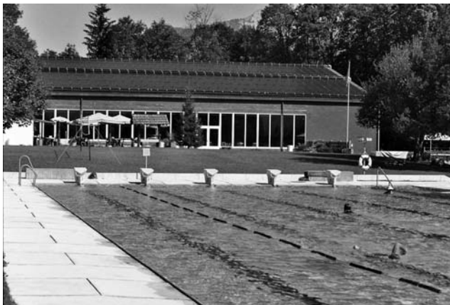
Solar water heating can work very well with swimming pools (Reproduced with permission from Energie Solaire)
