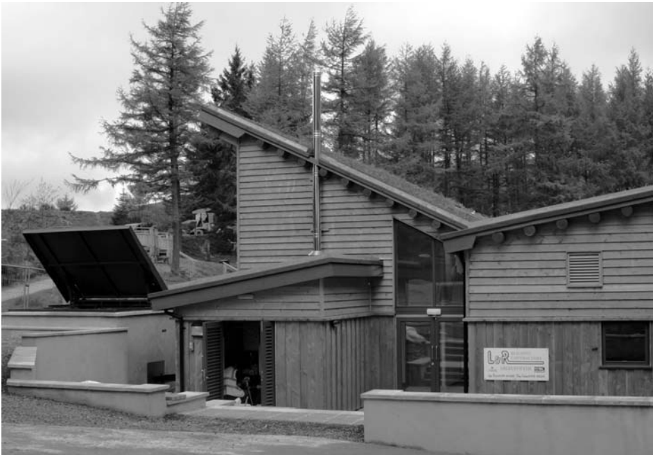
Space heating and hot water at the Nant y Arian Visitors Centre in Wales is provided by a 35 kW woodchip-fuelled boiler (Reproduced with permission from Dulas Ltd)
