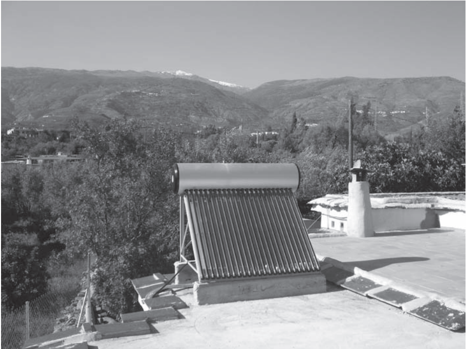
Integrated solar collector and header tank (Reproduced with permission from Powertech Solar)
