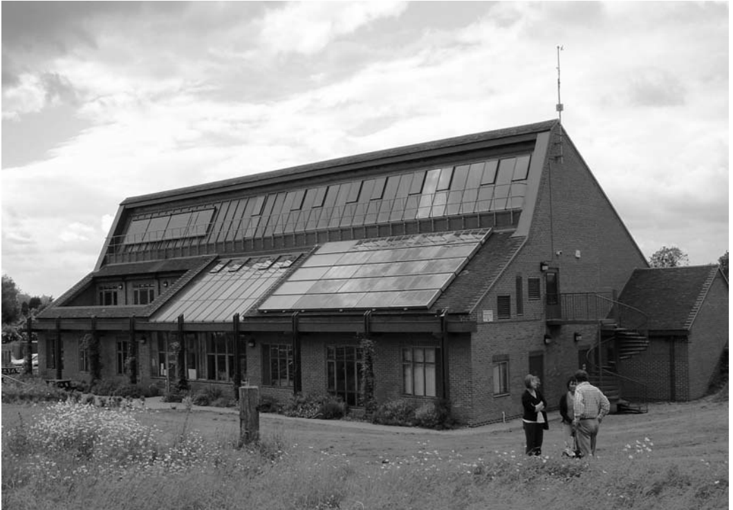
A super-insulated high thermal mass design was chosen for the Brocks Hill Environment Centre near Leicester, England. Solar PV, flat plate collectors and a 29kW wind turbine supply energy (Reproduced with permission from Henderson-Scott Architects)
