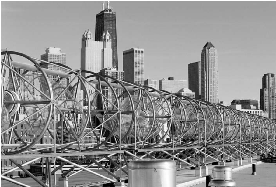
Development of building integrated wind turbines continues (Reproduced with permission from Kurt Holtz, Lucid Dreams Productions)
