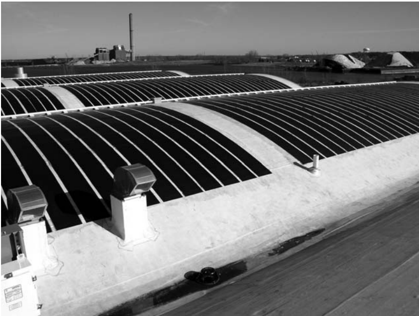
Roofing membranes incorporating PV cells open up new possibilities (Reproduced with permission from United Solar Ovonic)
