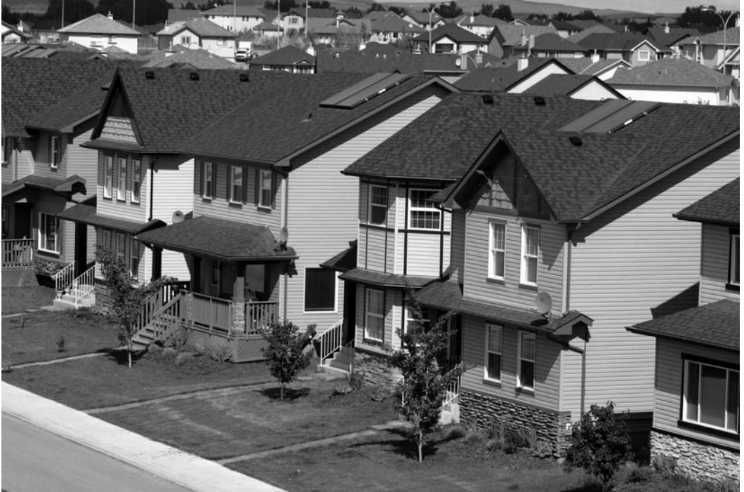
Houses on the development are popular with residents (Photo provided courtesy of Natural Resources Canada)
