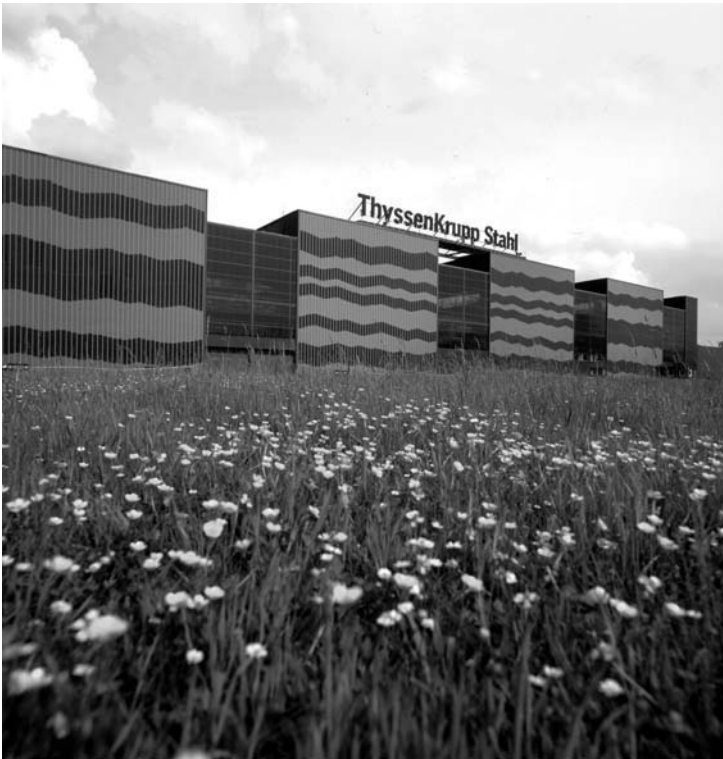
Façade mounted PV is a practical option in the right location (Reproduced with permission from United Solar Ovonics)
