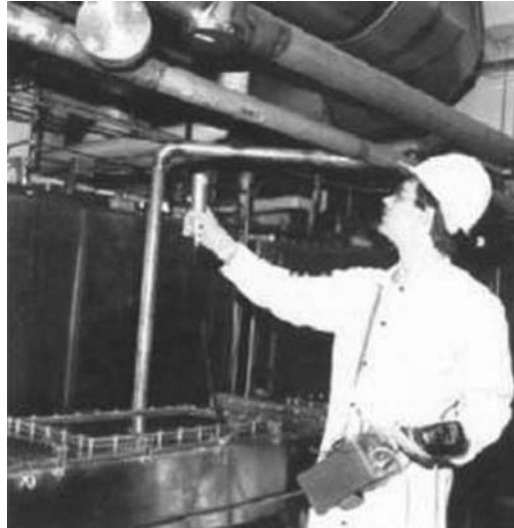
FIGURE 3C.3 GGH applied in a uranium facility to measure an overhead duct.
