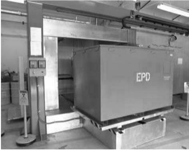
FIGURE 3A.22 The crated waste assay monitor (CWAM) installed at the Y-12 Plant, Oak Ridge, TN.
