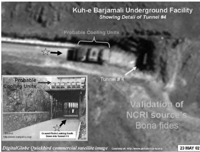
FIGURE 12.18 This figure is a closeup of the feature (believed to be cooling units on a framework) that is located outside the fourth tunnel (“Nuclear Tunnel”), compared with the ground photo provided by the Iran Policy Committee. (Sources: www.nci.org/05nci/09/nuclear%20tunnel.htm and www.globalsecurity.org/wmd/world/iran/images/dg_23may02_tehran-hemat_28.jpg .)
