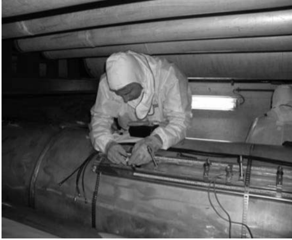
FIGURE 6.11 Flow sensor installation.
