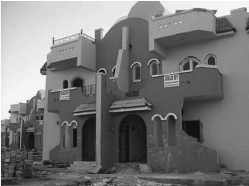
Figure 3.9 Second home under construction, Hurghada, Egypt
