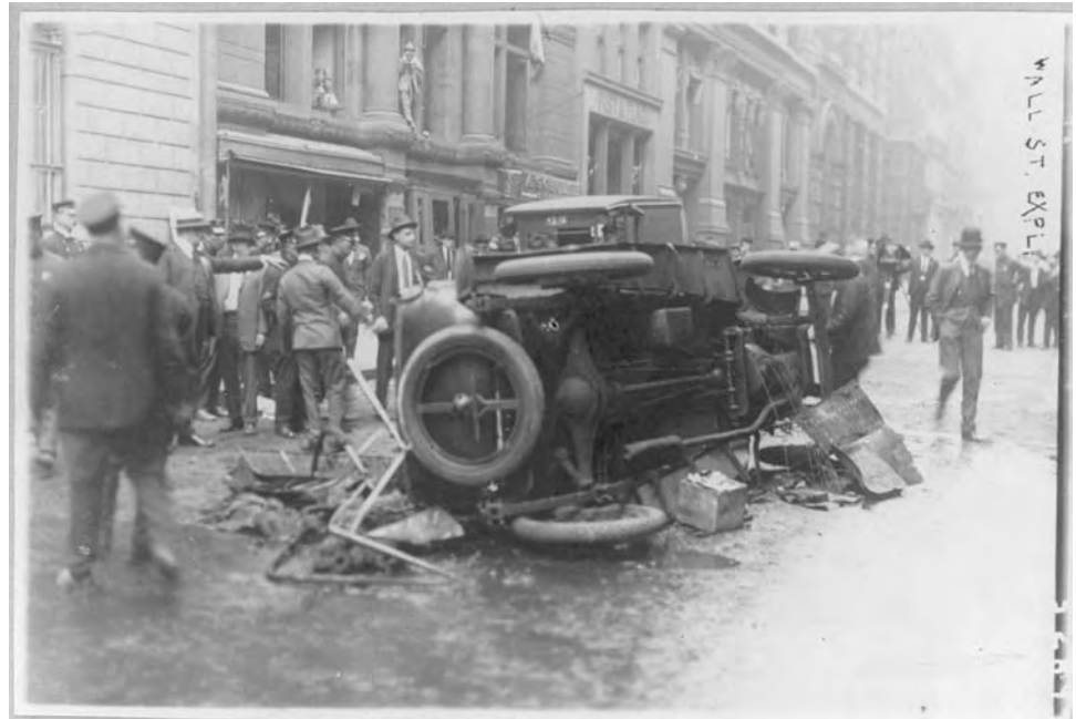
Wreckage from the Wall Street bombing of September 16, 1920
