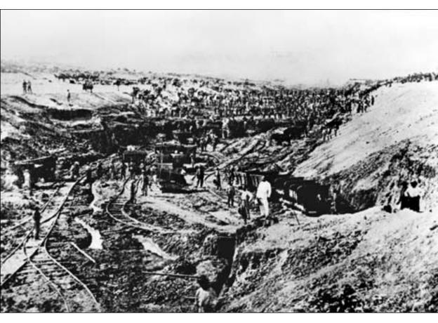
Construction on the Suez Canal began in 1859, and after 10 years of work, the canal opened for traffic on November 17, 1869. Workers are pictured here standing in the bed of the canal, which mostly passed through sand and alluvium.
