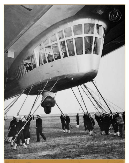
Landing the *Hindenburg* involved anchoring the dirigible to prevent it from floating away. As shown in this photo of a previous landing, the craft's crew dropped ropes during its descent, and men on the ground grabbed on and guided the ship to its resting spot.
