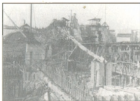
Work on the Panama Canal begins.
