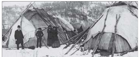
Mesquakie wigwams or lodges covered with reed (bulrush or cattail), photographed in wintertime at their settlement at Tama, IA, c.1890. (Photo Hudson's Gallery)
