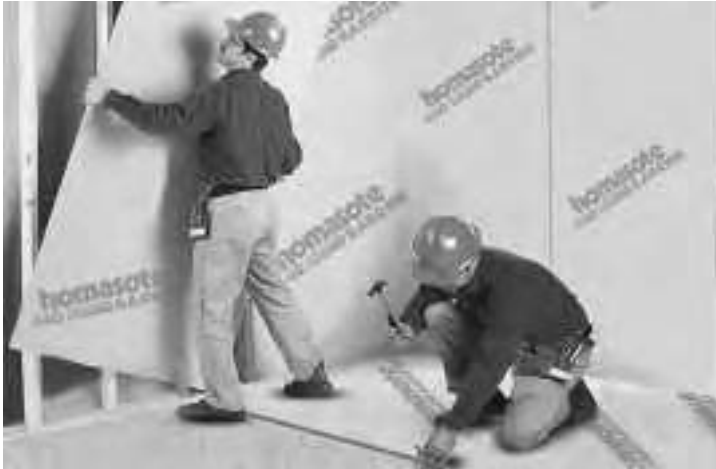
Homasote® panels from recycled newspaper installed in a building.
