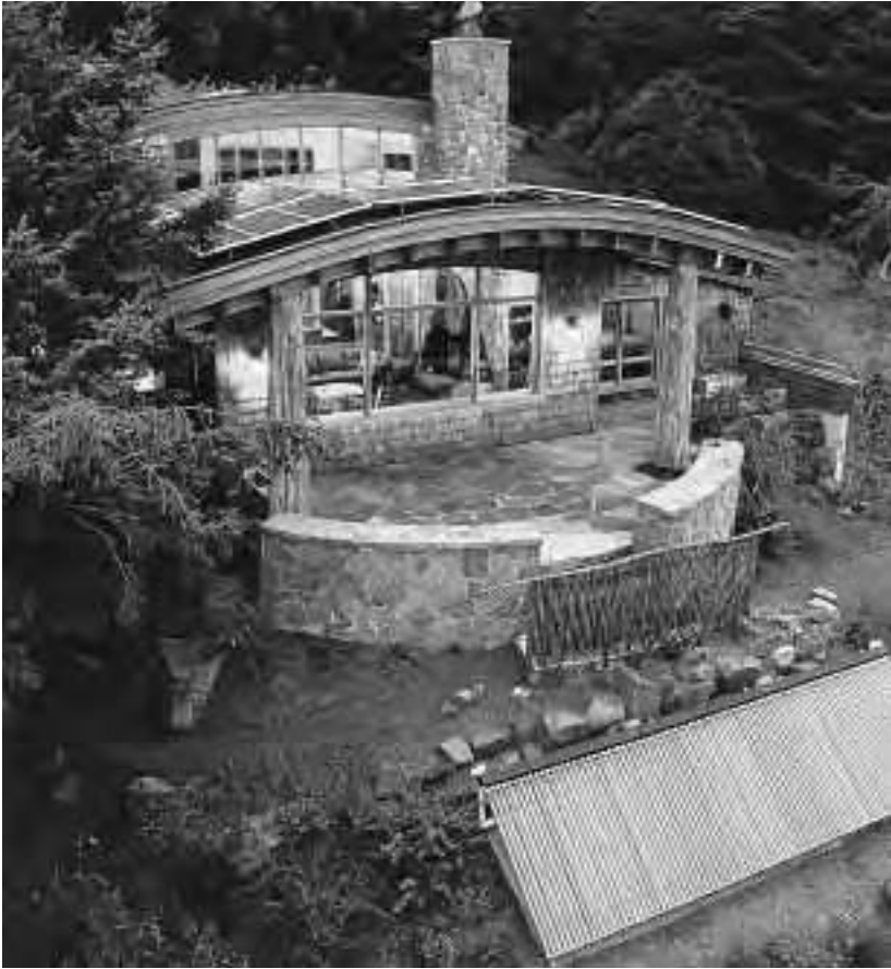
Photo by Dan Morrison, courtesy of Fine Homebuilding Magazine
