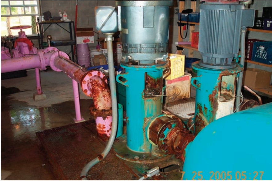
FIGURE 4 Accelerated corrosion by chlorine gas vapors resulting from recycled water being delivered directly into wet well of the pump station. Highly chlorinated recycled water should be delivered into open reservoirs to allow the corrosive vapors to release into the atmosphere (Tampa, FL).
