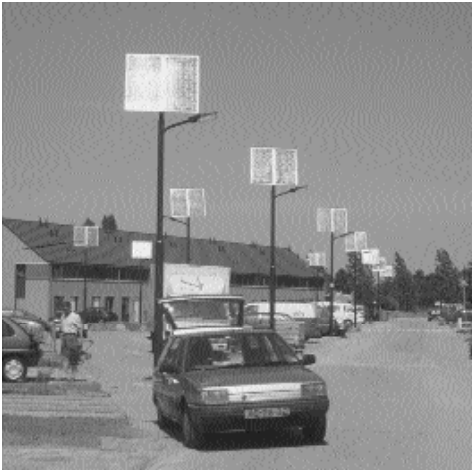
Solar-powered parking lot lights are seen here in a new ecological housing estate in Gouda, the Netherlands.
