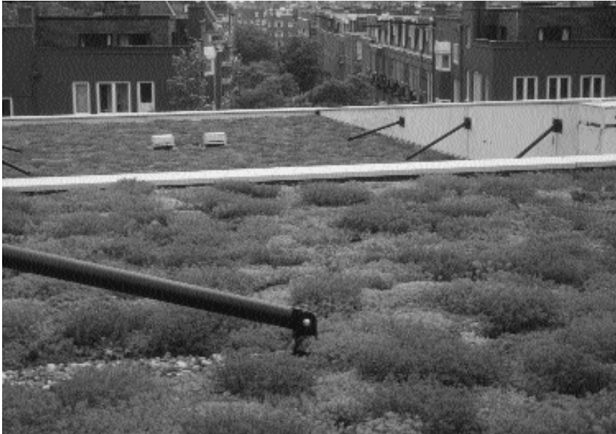
Greenroofs or eco-roofs are now common in Europe, especially in Germany, Austria, and the Netherlands. Shown here is a multilevel greenroof at the GWL-terrein housing complex in Amsterdam.
