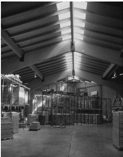
The Ecover ecological factory in Oostmalle, Belgium, incorporates many sustainable features, including extensive use of daylighting, as seen here.
