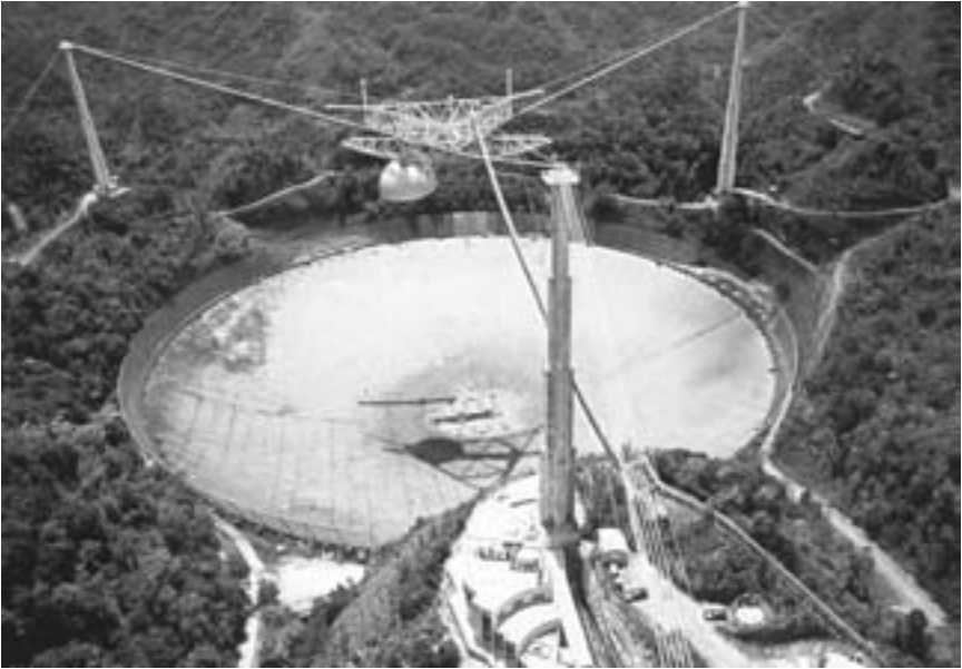
Figure 3.2. An aerial view of the 305-m-diameter Arecibo radio telescope in Puerto Rico. The observatory has a new visitor's center located in the lower part of the image; cars parked near the building give a sense of scale. Radio frequency receivers are located in the 900-ton platform suspended over the primary reflective surface. Arecibo Observatory is operated by the National Astronomy and Ionosphere Center (NAIC). Courtesy of the National Astronomy and Ionosphere Center.
