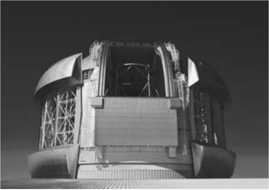
Figure 2.6. The Gemini North dome, shown here, is located in Mauna Kea, Hawaii, and was completed in 1998. The Gemini project is an international collaboration among the United States, the United Kingdom, Canada, Chile, Australia, Argentina, and Brazil that now operates two 8.1-m telescopes, one in each hemisphere. Gemini South is located at Cerro Pachón in Chile. The modern Gemini domes are constructed to almost “disappear” during observing, allowing air to flow around the telescope and keep it at ambient temperatures. Courtesy of the National Optical Astronomy Observatory, the Association of Universities for Research in Astronomy, and the National Science Foundation.
