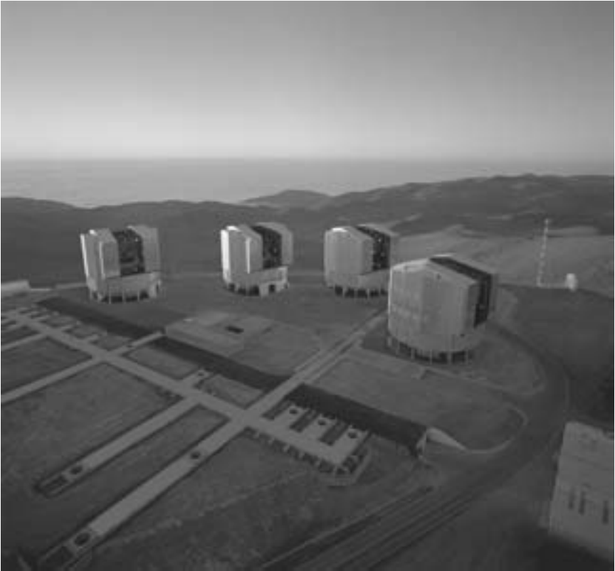
Figure 2.2. The European Southern Observatory (ESO) operates the Paranal Observatory in the Atacama Desert in northern Chile, seen here as photographed from the air. Paranal Observatory is the location of the four 8-m-diameter Unit Telescopes that have now been completed and seen first light. In combined mode, they have the sensitivity of a 16-m-diameter telescope. The concrete paths in the lower left corner of the image are tracks for three movable 1.8-m telescopes that will comprise part of the Very Large Telescope Interferometer (VLTi). Courtesy of the European Southern Observatory.
