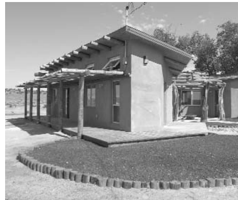
FIGURE 3.17. The builders of the Nageezi House in New Mexico attempted to incorporate salvaged wood whenever possible. Photo courtesy of ASU Stardust Center
