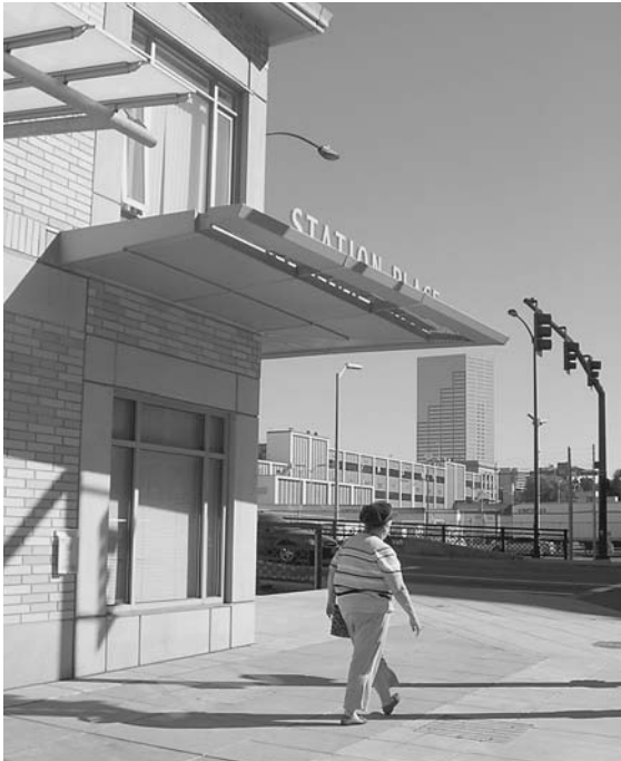
FIGURE 3.13. Station Place Tower in Portland, OR, includes an innovative strategy for using rainwater captured from the roof.
