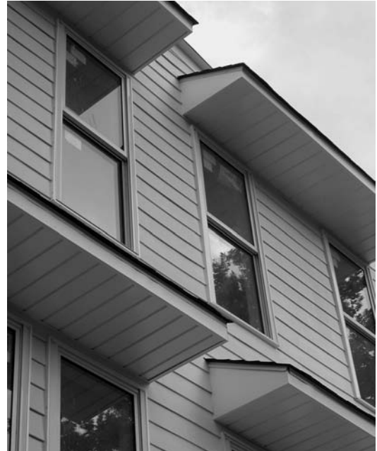
FIGURE 3.6. Window overhangs, such as these on the Bellevue Court project in Trenton, NJ, can be a design element while also providing shading to cool a building.
