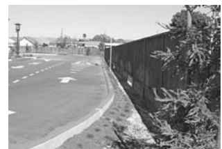
FIGURE 3.3. The bioswale system at Nuevo Amenercer helps improve the quality of water draining off the site.
