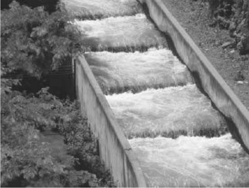
Figure 5.1. Fish Ladder at Rocky Reach Dam, Washington (Photograph by Frank R. Spellman)
