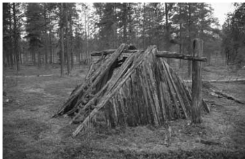
Fig. 2.4. Sami hut dwelling, Rebraure, Arjeplog parish, Sweden. The hut was probably built in the 19th century and abandoned in the early 20th century. This type of log construction is typical of the forest Sami in the Arjeplog, Jokkmokk and Arvidsjaur areas. Photo by Lars Liedgren.
