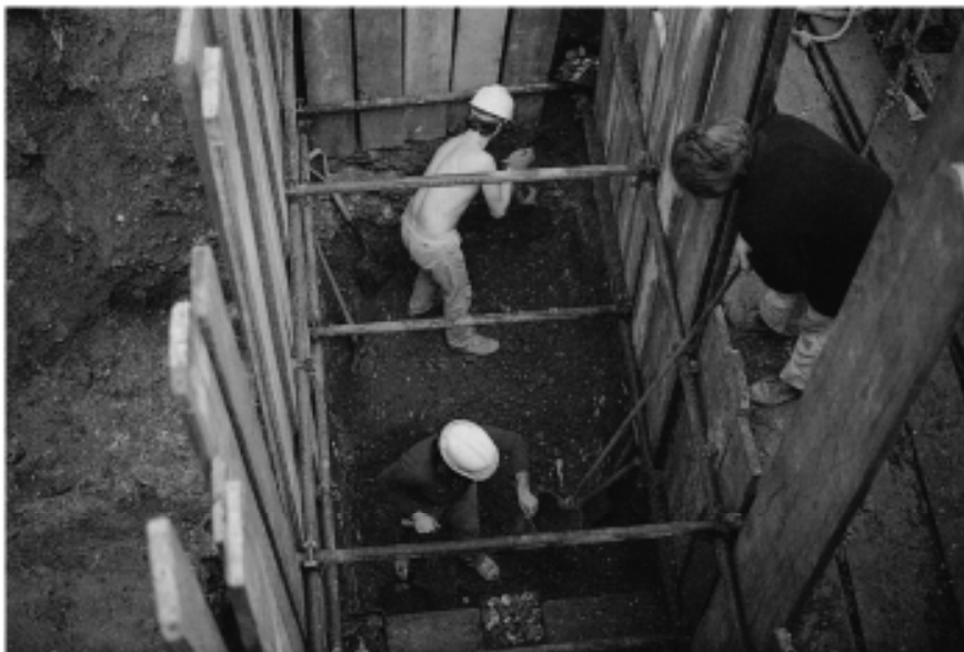
Figure 5.2 Site safety: shoring of a narrow trench.
