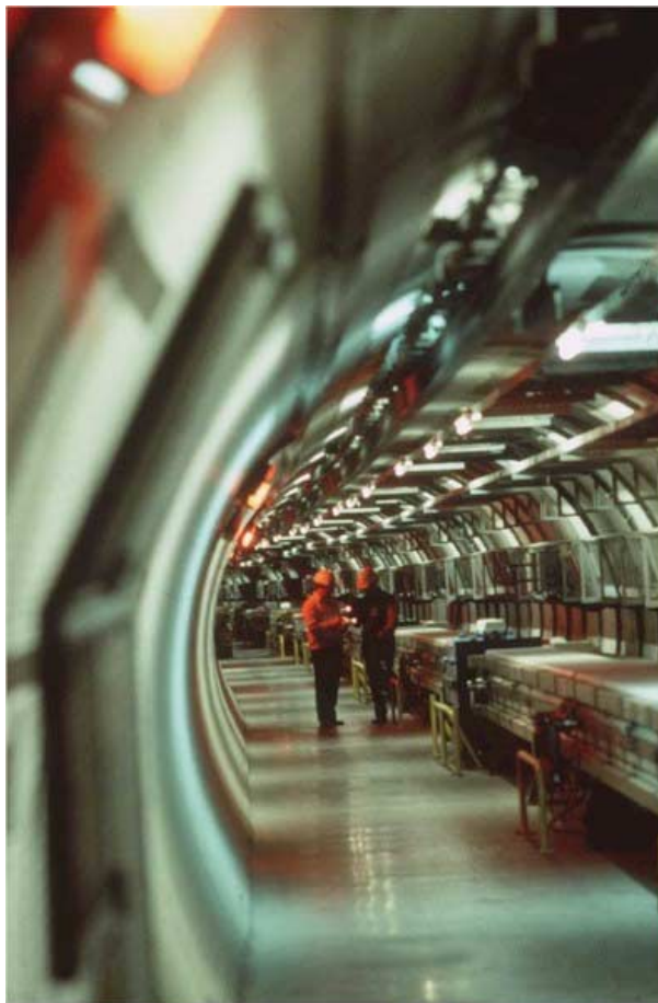
Fig. 4.10. A cross section of the LEP accelerator ring at CERN, Geneva. The ring is 5 miles in diameter and the tide of the Moon causes this to stretch and shrink daily by as much as 1 millimeter, as can be sensed by the accuracy of the detectors used in experiments (Figure 5.4).
