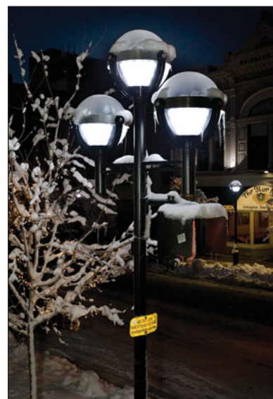
▲ FIGURE 1.22 LED lighting. Ann Arbor, Michigan, has replaced incandescent streetlights with white LEDs. The city estimates the change will save $100,000 per year and reduce annual greenhouse gas emissions by 267 tons.
