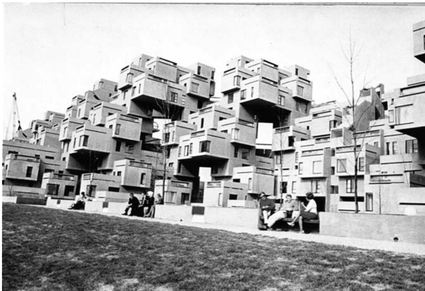
Figure 4.23 Moshe Safdie, Habitat 67 ( Habitat '67 ). Individual cells or units assembled into a residential community for the 1967 Expo in Montreal. In Michel Ragon, La cité de l'an 2000 . Courtesy of Éditeur Casterman.
