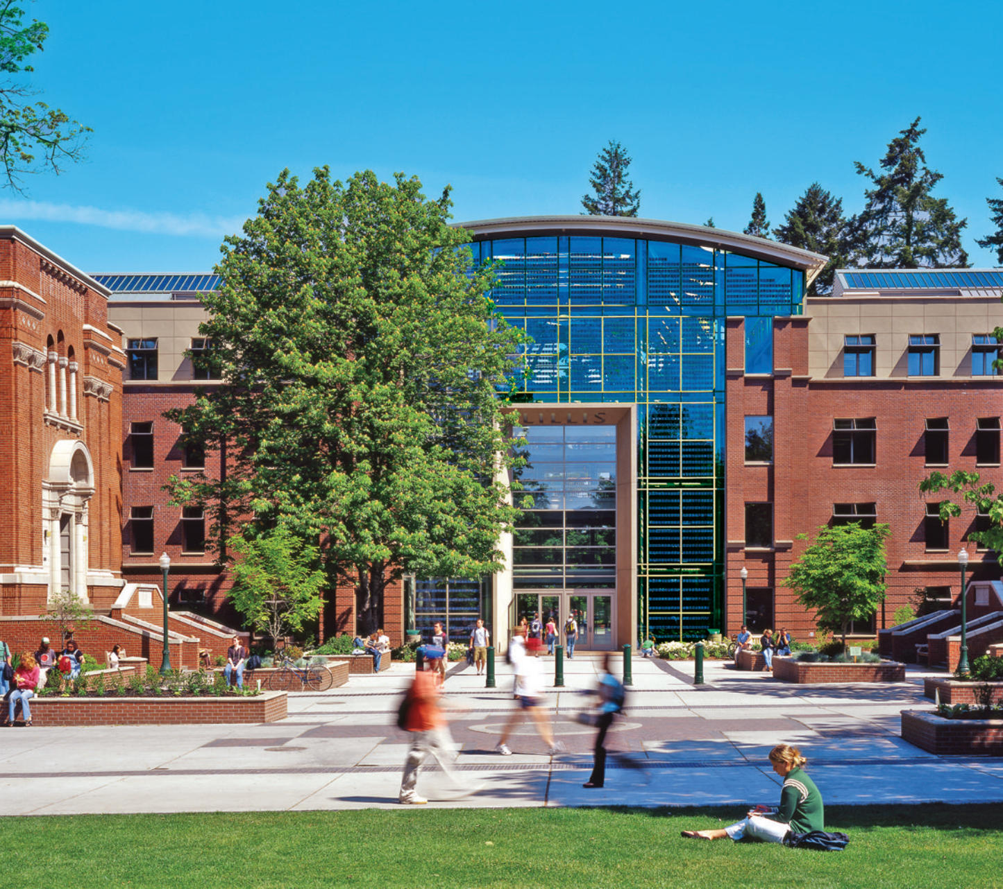
Figure C-22 The Lillis Business Complex at the University of Oregon creates a bridge between the older business buildings while providing daylight to lecture rooms and interior spaces via glazing with integrated photovoltaic cells embedded in the central atrium's glass. (Architect: SRG Partnership) Image © Lara Swimmer.
