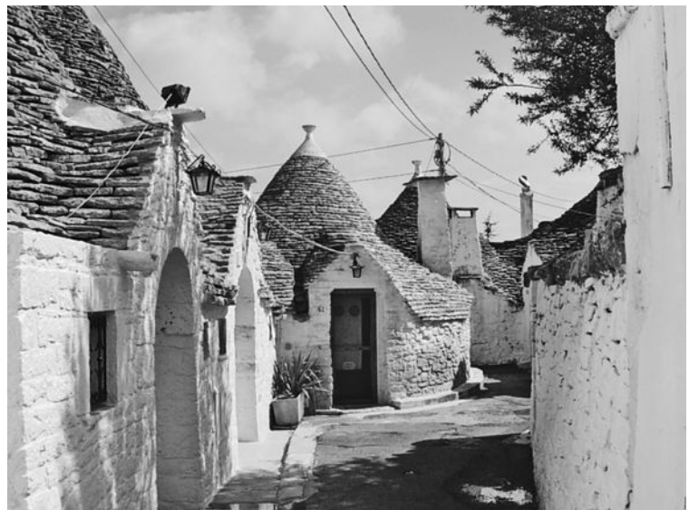
► Figure 1-4 The town of Alberobello, a UNESCO World Heritage site, contains an urban concentration of more than 1,500 Trulli dwellings, dating from the mid-fourteenth century that are still in use and were made from limestone blocks collected from surrounding fields. These indigenous structures could be quickly erected and dismantled, utilizing ancient mortarless drystone construction for their distinctive conical roofs that draw off the heat of their southern Italian climate. Image courtesy of John Boecker.
