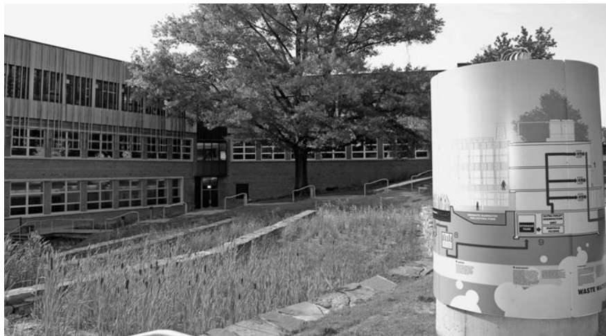
Figure 6-3 The completed constructed wetland at the Sidwell Friends School cost less than connecting to the municipal sewer system. Image courtesy of Sidwell Friends.
