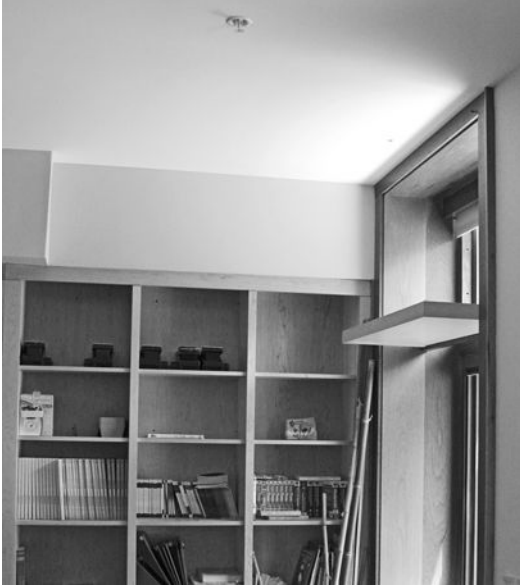
Figure 6-21 Interior light shelves reflect daylight that enters through the upper section of window glass deeper into the space. This portion of glass above the light shelf is selected for its daylighting properties and has a higher visible light transmittance than the vision glazing below. Image courtesy of Todd Reed.
