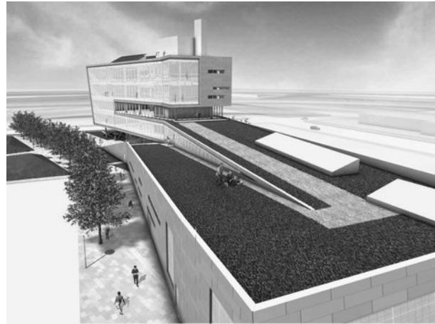
Figure 6-39 Renderings of the proposed Syracuse Center of Excellence project, which is pursuing LEED Platinum certification, depict south-facing glazed walls (image on the right) for this cold climate along with extensive green roofs. Images courtesy of Toshiko Mori Architect.
