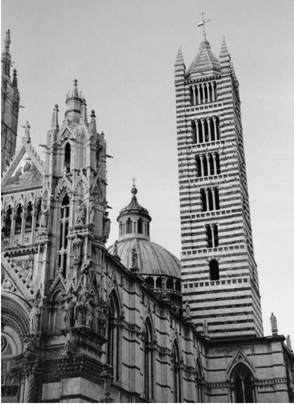
Figure 1-9 The striking Romanesque marble banding of the Siena Duomo's campanile (bell tower), which was added in 1313, extends the pattern of the cathedral's exterior materials. Almost all of the marble used for the cathedral was harvested by inhabitants of the town from local quarries. Image courtesy of John Boecker.
