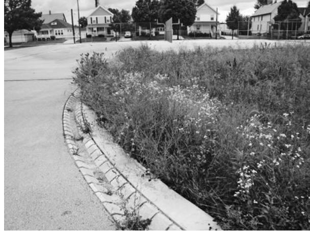
Figure 6-27 This rain garden captures and infiltrates the rainwater runoff from the adjacent paved surfaces via slotted gutters. Image © 2008 Conservation Design Forum, Elmhurst, IL, http://www.cdfinc.com .
