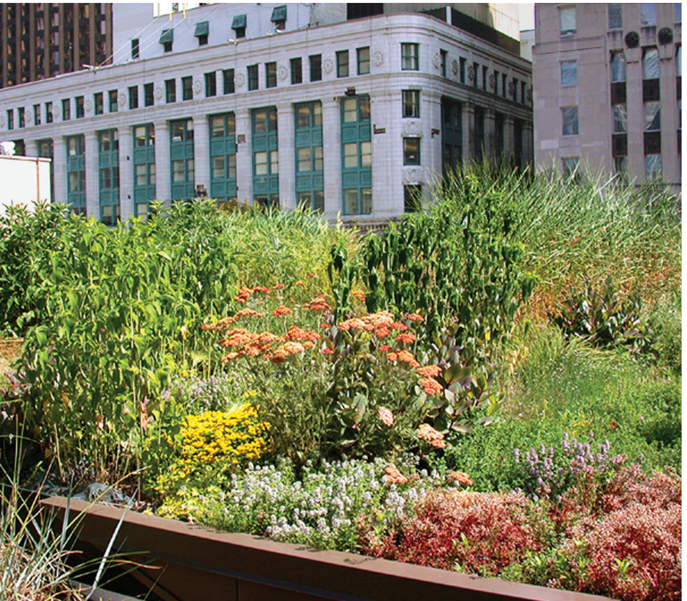
Figure C-12 Chicago's City Hall was renovated with an extensive vegetated roof garden, completed in 2001, that covers more than 20,000 square feet of roof area. Effects associated with this vegetated roof decreased annual utility bills by $5,000. Image © Conservation Design Forum, Elmhurst, IL, www.cdfinc.com .
