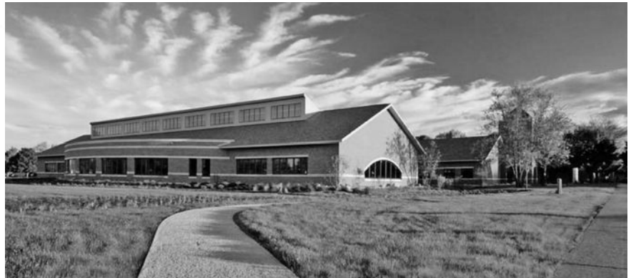
▶ Figure 6-14 The finished library at the Associated Mennonite Biblical Seminary in Elkhart, Indiana. Image courtesy of DJ Construction.
