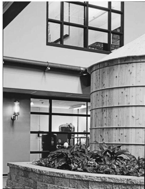
Figure 7-11 Harvested rainwater stored in the cistern at DEP's Norristown, Pennsylvania facility satisfies 100 percent of the building's annual toilet-flushing demand. The system's sediment filter and pumps are housed in an adjacent room behind a glass partition as a means of educating visitors about the system. Image ©2004 Jim Schafer.
