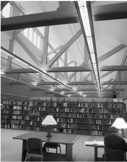
Figure 6-23 These clerestory windows at the AMBS project provide effective toplight daylighting for producing even illumination within the library space. Image courtesy of Marcus Sheffer.
