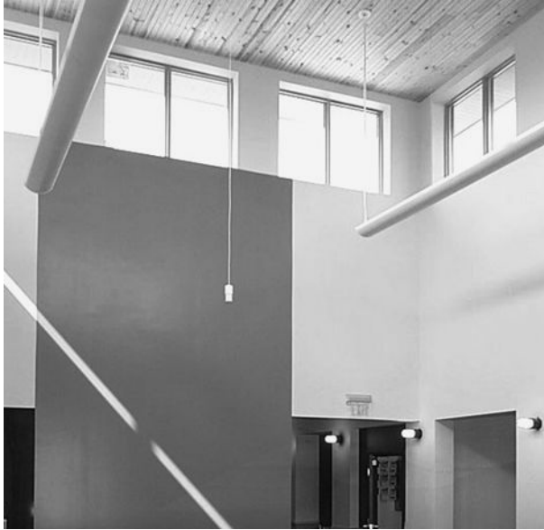
▲ Figure 6-25 These clerestory roof monitors bring copious daylight into the main map room of the DEP Cambria project from all four directions, allowing for the photocell sensor (center) to fully dim the lighting fixtures during most daylight hours. This toplighting strategy is often used to illuminate common areas such as lobbies. Image courtesy of John Boecker.
