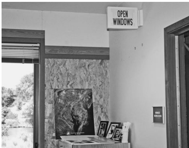
Figure 4-2 The Chesapeake Bay Foundation Headquarters, Annapolis, Maryland, design team resolved the dilemma between HVAC efficiency and operable windows by installing sensors and controls that shut down the mechanical system and light a sign instructing occupants to “open windows” when outside air temperature and humidity conditions are appropriate. Image courtesy of Marcus Sheffer.
