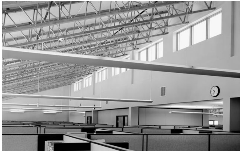
Figure 6-24 The north-facing clerestory windows at the DEP Cambria, Pennsylvania, project provide bilateral daylighting to create balanced lighting-level distributions in this open office space; punched openings on the opposite lower wall (not depicted) introduce daylight into the same space from the south. Image ©2000 Jim Shafer.
