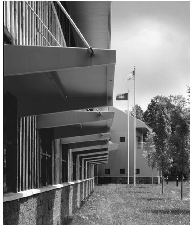
Figure 2-6 Light shelves at south-facing windows of the Pennsylvania DEP Cambria project shade windows below from high-altitude solar radiation in the summer while allowing low-altitude winter sun to penetrate; they also bounce daylight deeper into interior spaces through the glass directly above the light shelves, reducing the need for artificial lighting. Copyright © Jim Schafer.
