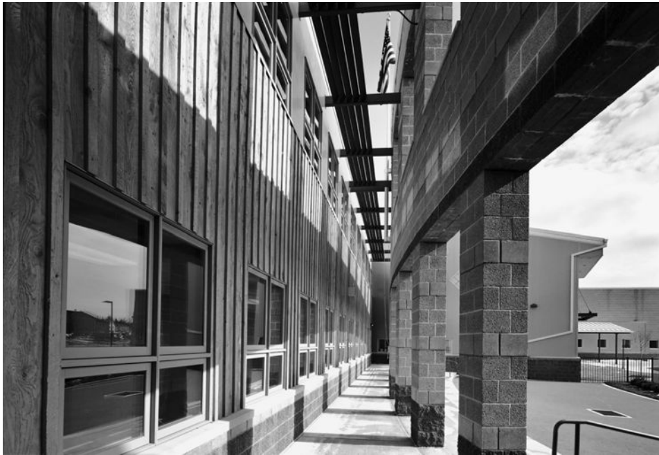
Figure 7-16 The Clearview Elementary School in Hanover, Pennsylvania, also incorporated local indigenous hemlock siding; in addition to its environmental benefits, it reflects the local, agricultural, and rural architectural context of century-old wood barns in nearby surrounding areas. Image ©2003 Jim Schafer.
