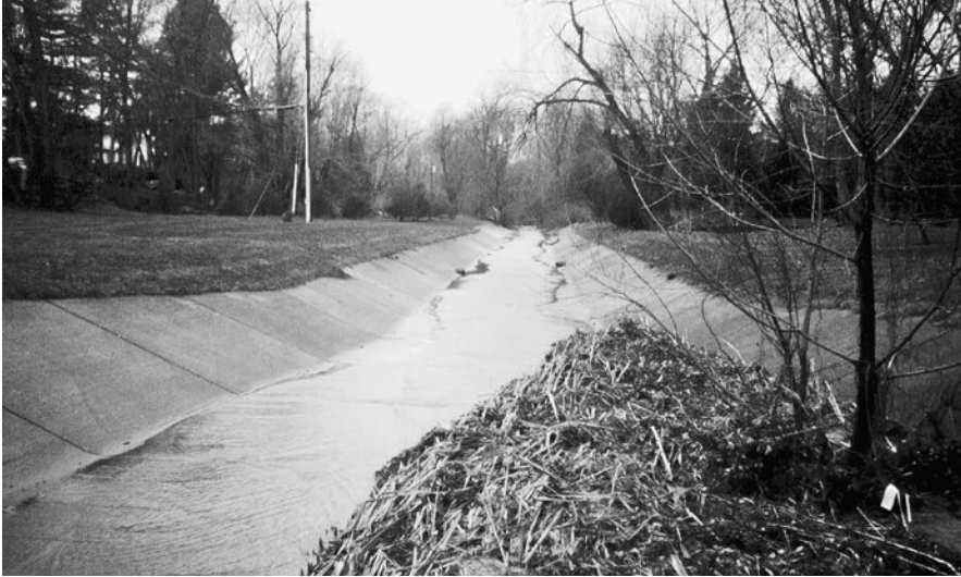
Figure 3-11 The original “concrete stream,” stormwater conveyance system solution for a site in Baltimore, Maryland. Image courtesy of Biohabitats, Inc.
