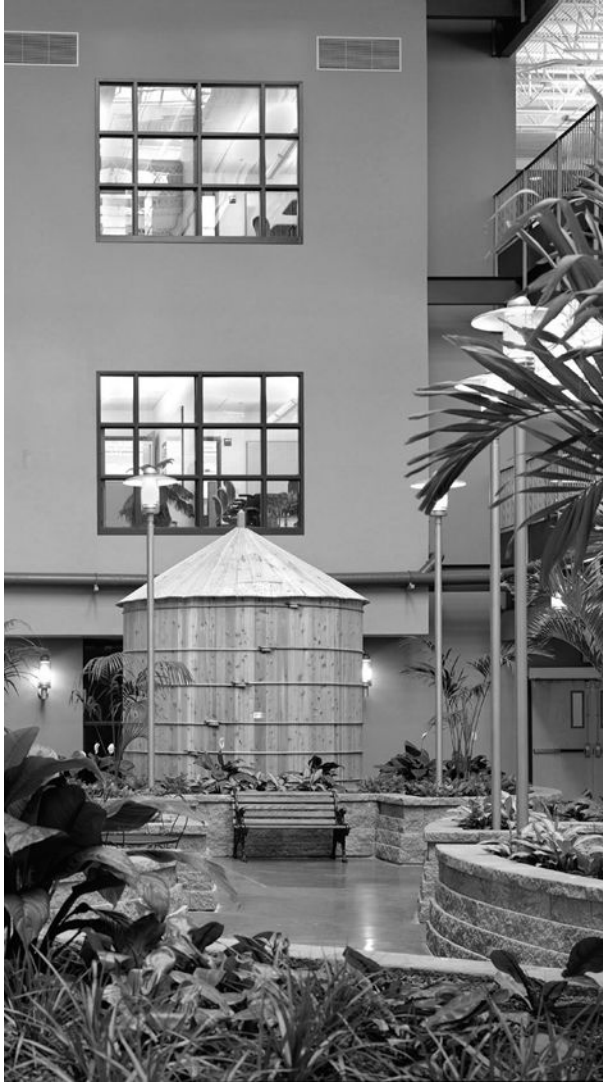
Figure 4-15 In the DEP Southeast Regional Headquarters building in Norristown, Pennsylvania, rainwater is collected and stored in a cistern, located in the building's atrium, that is fed by exposed piping from the roof. A sediment filter and pump used to convey this harvested rainwater for flushing toilets (satisfying 100 percent of the building's toilet-flushing demand) are located in an adjacent room behind a glass partition, so that the entire system is visible to visitors as a means of providing education about rainwater harvesting (see Figure 7-11). Image © Jim Schafer.
