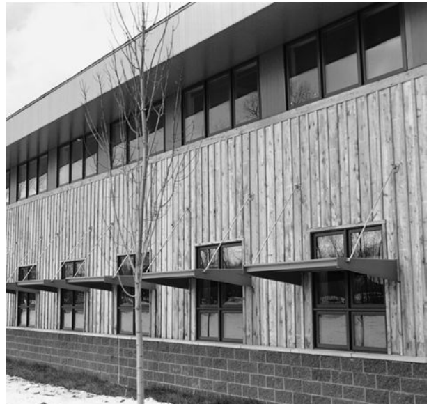
Figure 7-15 Unpainted, locally harvested hemlock siding at the DEP Cambria, Pennsylvania, building significantly reduced costs and environmental impacts; its board and batten installation allows it to dry while on the building, thereby reducing the embodied energy and emissions associated with typical kiln drying. Image ©2001 Jim Schater.
