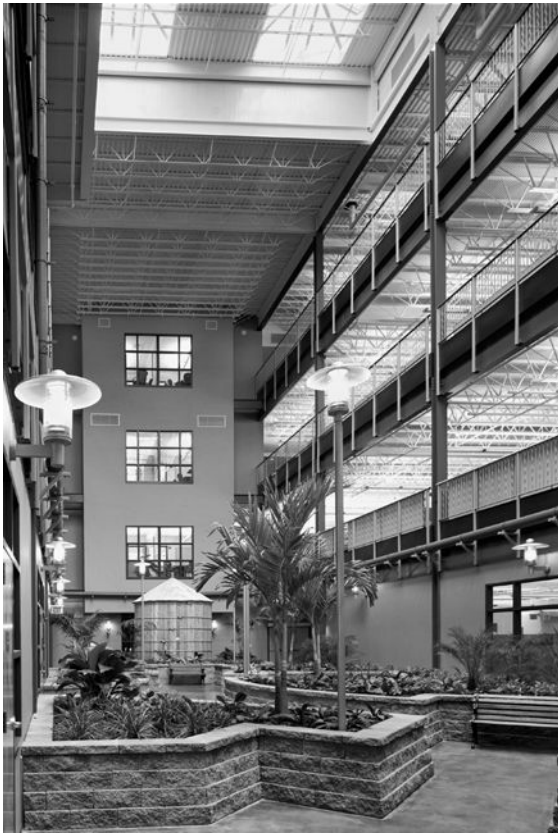
▲ Figure 7-12 The rainwater-harvesting cistern of the DEP Norristown project is located in the building's atrium and also supplies water to a hose bib for watering atrium plants. Image ©2004 Jim Schafer.
