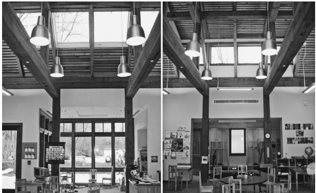
▲ Figure 6-25 These clerestory roof monitors bring copious daylight into the main map room of the DEP Cambria project from all four directions, allowing for the photocell sensor (center) to fully dim the lighting fixtures during most daylight hours. This toplighting strategy is often used to illuminate common areas such as lobbies. Image courtesy of John Boecker.
