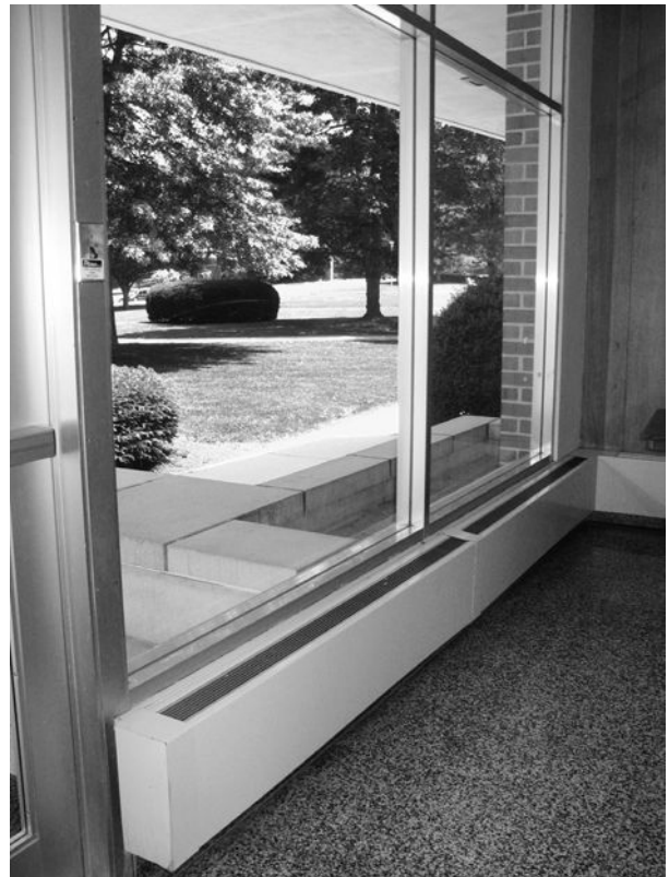
▲ Figure 2-7 High-performance windows—like this triple-glazed, aluminum-clad, wood window—reduce heat loss and can eliminate the need for perimeter heating systems. Image courtesy of Loewen. Copyright © C. P. Loewen Enterprises Ltd.
