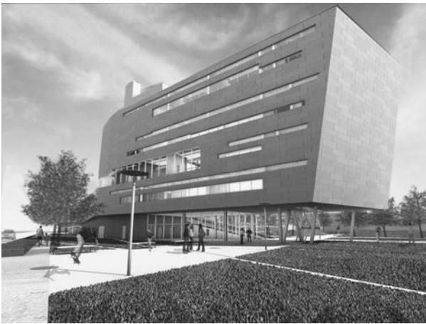
Figure 6-39 Renderings of the proposed Syracuse Center of Excellence project, which is pursuing LEED Platinum certification, depict south-facing glazed walls (image on the right) for this cold climate along with extensive green roofs. Images courtesy of Toshiko Mori Architect.
