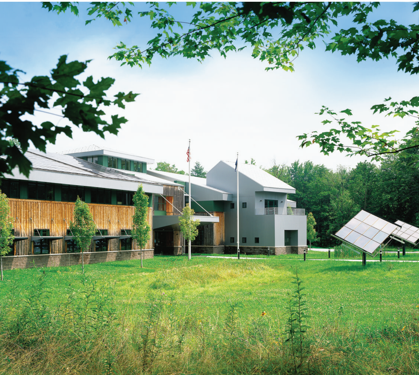
Figure C-17 The Pennsylvania Department of Environmental Protection's Cambria office building in Ebensburg, Pennsylvania, includes south-facing light shelves, rooftop solar panels, and a pair of photovoltaic trackers flanking the entrance walk. (Architect: Kulp Boecker Architects) Image © Jim Schafer.
