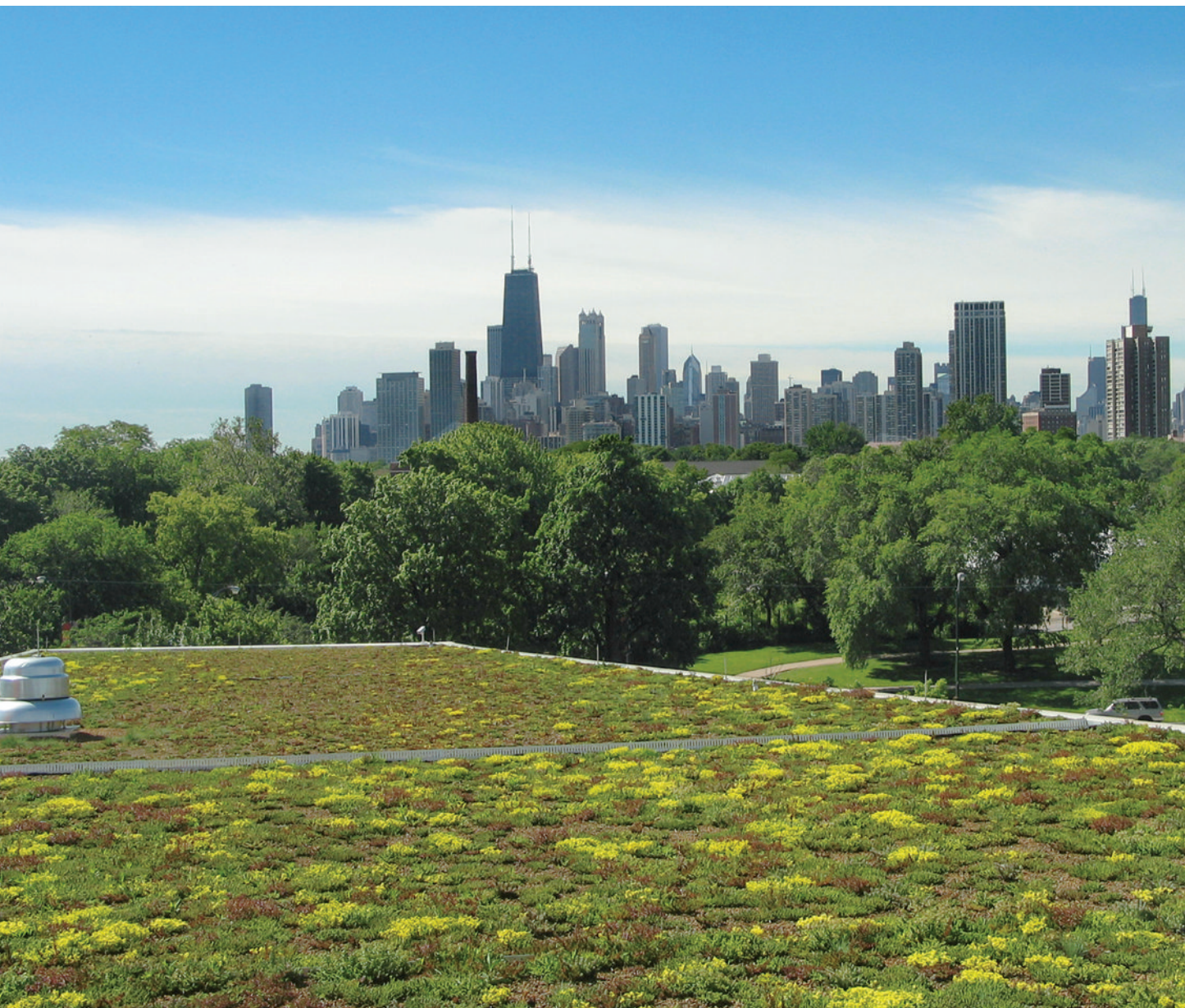
Figure C-13 This vegetated roof on the Peggy Notebaert Nature Museum creates a beautiful landscape in Lincoln Park, Chicago. Design guidelines for green roofs can be found at www.naturemuseum.org/greenroof/planningarroof.html (accessed January 2009). Image © Conservation Design Forum, Elmhurst, IL, www.cdfinc.com .
