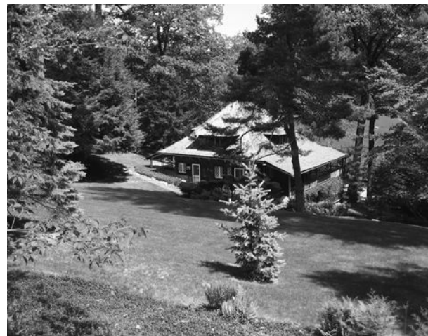
Figure 1-15 A cabin with a fireplace in the Adirondacks is free from any HVAC problems. Image courtesy of Todd McFeely.
