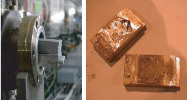
Figure 3.17 The power of wiggler radiation. These images of a runaway failure of the beam-defining aperture in the front end of a wiggler beamline at the Swiss Light Source demonstrate the power delivered at synchrotron facilities. The aperture consists of two pairs of tungsten blocks, and is (or, rather, was) the first component in the beamline, and therefore ‘sees’ the full spectrum of radiation from the wiggler. This includes the soft x-ray component, which is very efficiently absorbed by matter, before this dangerous spectral component is removed by a carbon or diamond filter. Failure occurred because the upper block was not held sufficiently firmly in place, and dropped marginally into the beam path. The increased heat load caused the support structure, made of copper, to also become hot, which loosened further and allowed the W-block to sag more . . . resulting in a runaway failure. The entire beam became occluded and the upper block became so hot that the two steel M8 screws at the front evaporated, and the upper and lower W-blocks fused together. The absorbed power was over 8 kW. Note that the boiling point of iron is 3134 K, while the melting point of tungsten is 3695 K!
