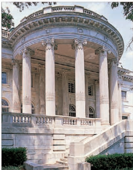
South portico of the DAR Memorial Continental Hall
