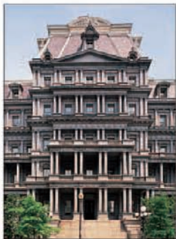
Imposing façade of Eisenhower Old Executive Office Building
