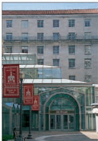
The Old Post Office Pavilion
