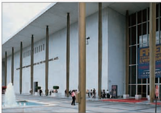
Façade of the John F. Kennedy Center for the Performing Arts
