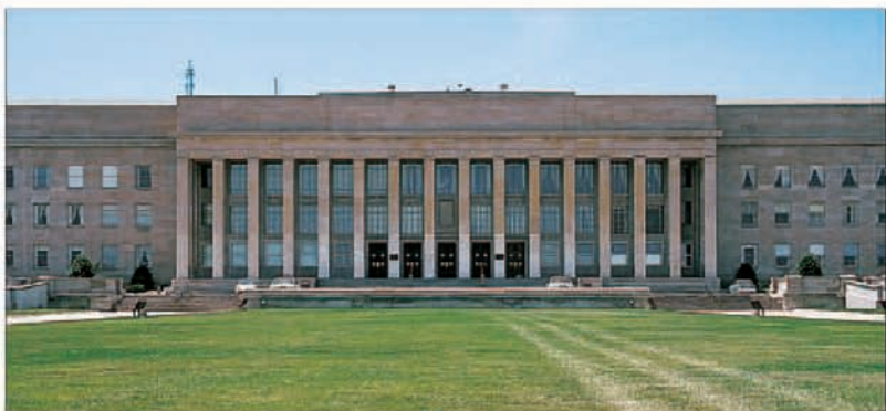
View of the Pentagon building's formidable concrete façade from the Potomac River
