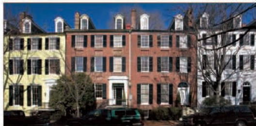
Smith Row, American Federal-style architecture on N Street ⑪
