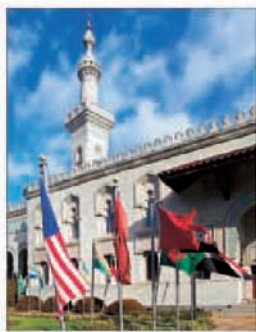
Islamic Center's striking minaret ⑦
