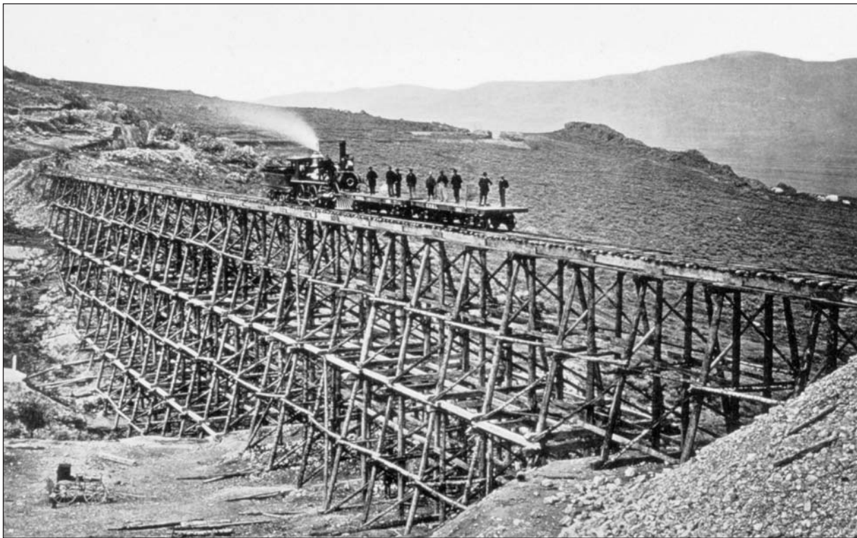
Construction workers for the Central Pacific Railroad stand on flatcars near Promontory Point in 1868, a year before the transcontinental railroad was completed. The opening of this railroad generated millions of dollars for the “big four” owners of the Central Pacific—Charles Crocker, Mark Hopkins, Collis P. Huntington, and Leland Stanford. (Library of Congress)
