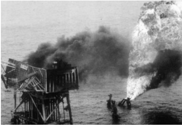
11.6 Piper Alpha destroyed.
