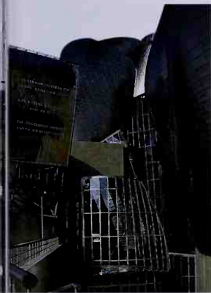
The Guggenheim Museum in Bilbao, Spain (1998), by Frank Gehry.
