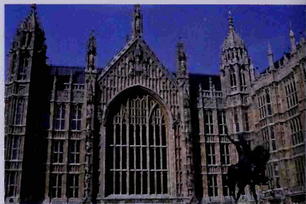
Barry's Westminster New Palace, London (1836-68) —the Houses of Parliament to you and me—is the first significant Gothic Revival building. The authentic Gothic detail was provided by A.W.N. Pugin.
