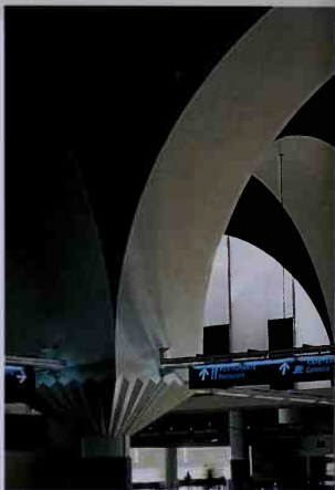
The arches of the airport buildings in Seville by José Rafael Moneo are characteristically Moorish features.
