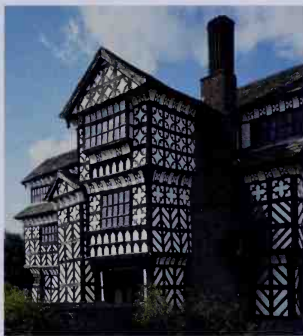
Little Mareton Hall, Cheshire (1550-59), a typical Tudor courtier's home, manages to house a long gallery. Timber framing is put to ornamental use (same call this early Renaissance).
