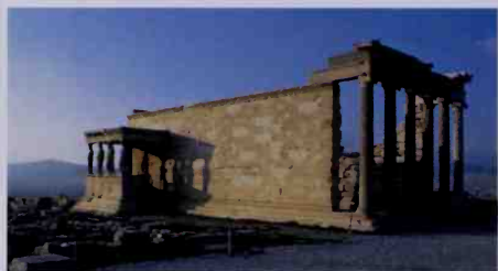
The Ionic Erechtheion (421–406 B.C.) on the Acropolis replaced the temple of Athena destroyed during the Persian invasion. Caryatids support the roof over the porch on the south façade.
