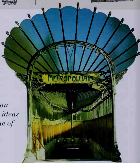
The entrance to the Porte Dauphine metro station in Paris (c.1900) is typical of the arresting Art Nouveau designs of Hector Guimard.
