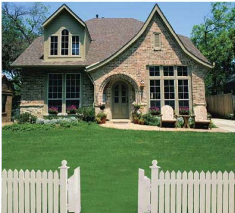
These two properties have spacious Bright Halls in front of the Main Door, enabling Qi to collect in front of the house.
