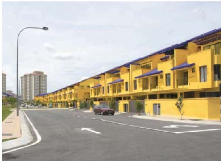
Lamp post directly in front of Main Door.
