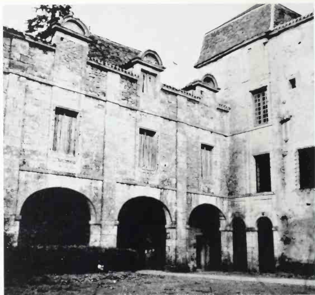
421 Génovévain Priory of Saint-Jean-de-Côle. Monastic buildings, c. 1600.
