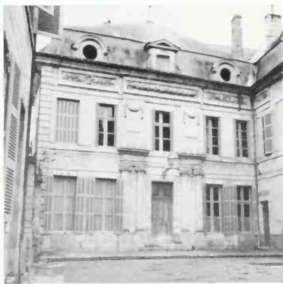
486 Abbey of Fontevault. Abbess's lodging, c. 1775.
