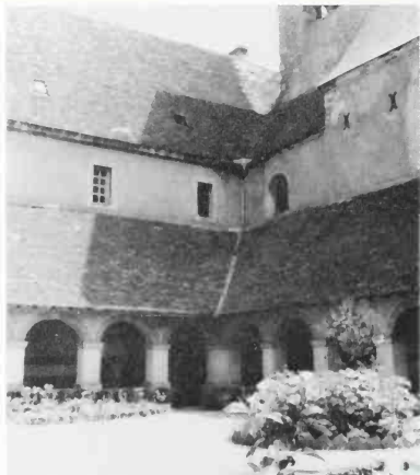
707 Minimes of Decize. Cloister, c. 1600.
