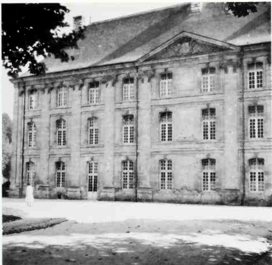
515 Abbey of Prémontré. Northern wing of west block, c. 1720.
