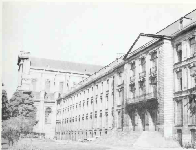
256 Benedictine Abbey of Saint-Vaast, Arras. Monastic buildings by Contant d'Ivry, 1746. West façade.
