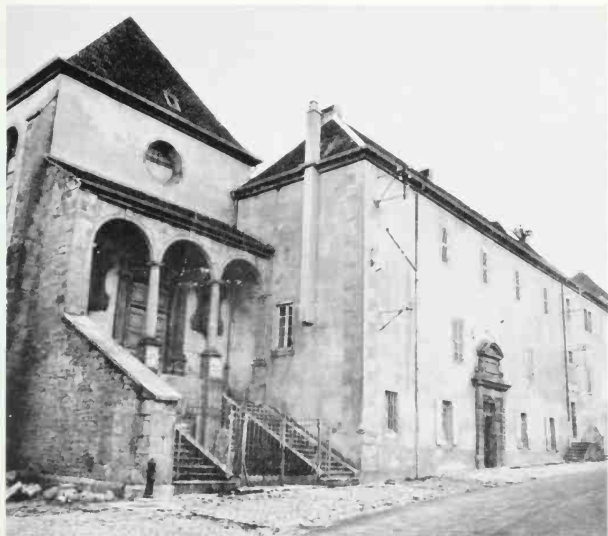
354 Cistercian Nunnery, Orgelet. By Dom Vincent Duchesne, 1708-18. Exterior.
