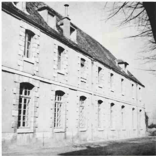
664 Cordeliers of Chartres. Monastic buildings, c. 1630.
