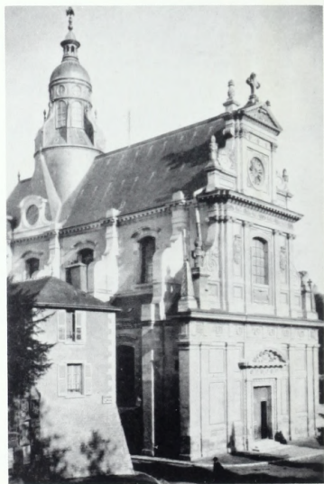
735 Jesuit College of Saint-Louis (now Saint-Vincent-de-Paul), Blois. Façade, by Martellange, 1625.
