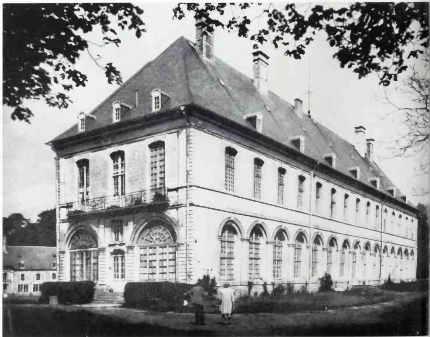
380 Cistercian Abbey of Cercamp. Main block, south, c. 1740.
