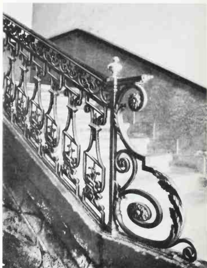
743 Jesuit Maison Professe, Paris. By Martellange and Derand, 1627-41. Staircase.
