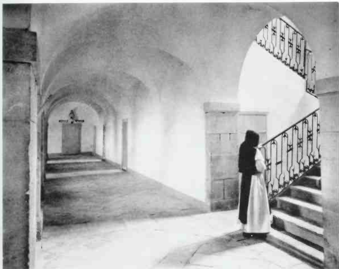
370 Cistercian Abbey of La Grâce-Dieu. Passage to the cells, 1720-6.
