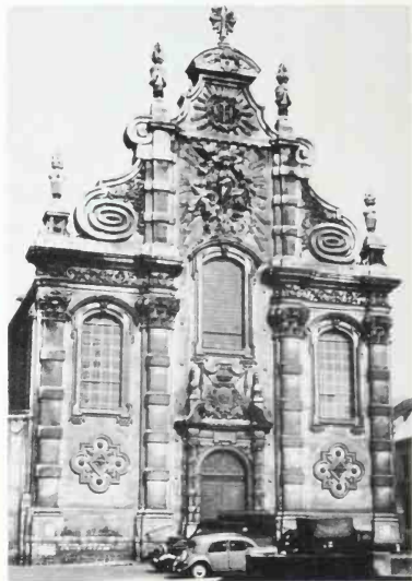
761 Jesuits of Cambrai. Façade of chapel, 1692.
