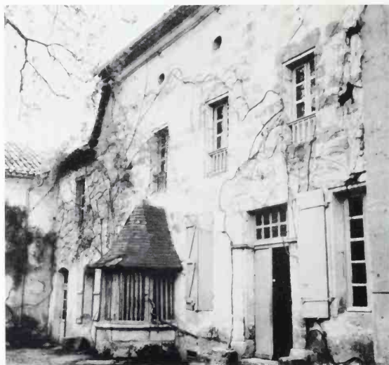
676 Convent of Clarisses, Aubeterre. 1608. Courtyard.
