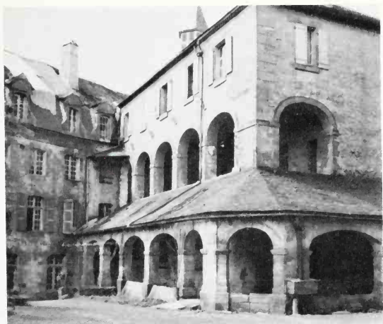
677 Convent of Clarisses, Sarlat. Cloister, c. 1650.
