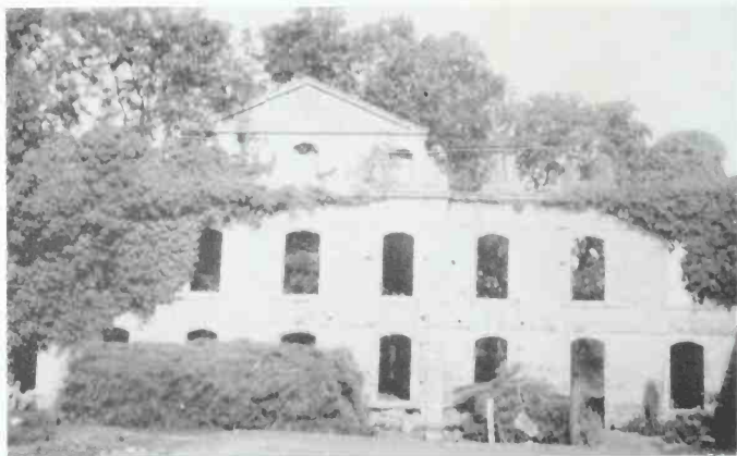
369 Cistercian Abbey of Coët-Malouen. Ruins of monastic buildings, 1709.
