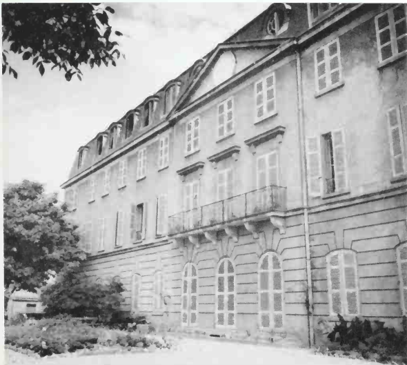
658 Dominicans of Poligny. Monastic buildings, by Amondry, 1715.
