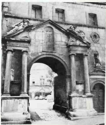
672 Cordeliers of Dôle. 1737-47. Entrance.
