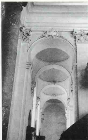
774 Jesuit Church of Saint Pierre Colmar. 1742-50. Aisle.
