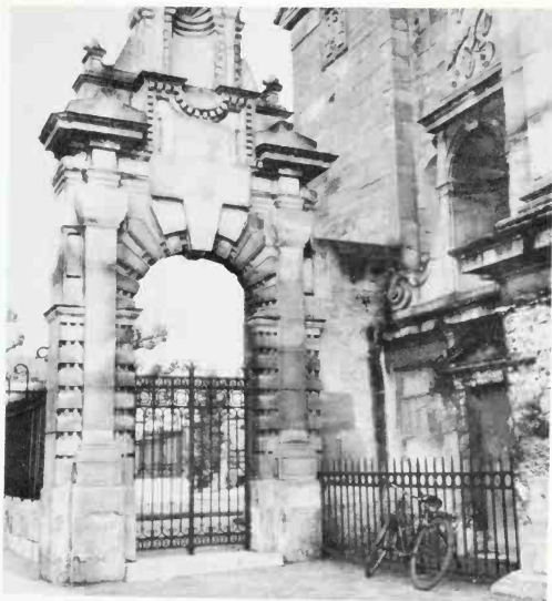
585 Saint-Bruno, Bordeaux. 1665. Entrance of the former convent.
