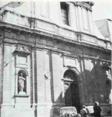
Jesuit College, Montpellier. Chapel, now Notre-Dame-des-Tables, by Jean Giral and Frère Monestier, 1707-48. Side.
