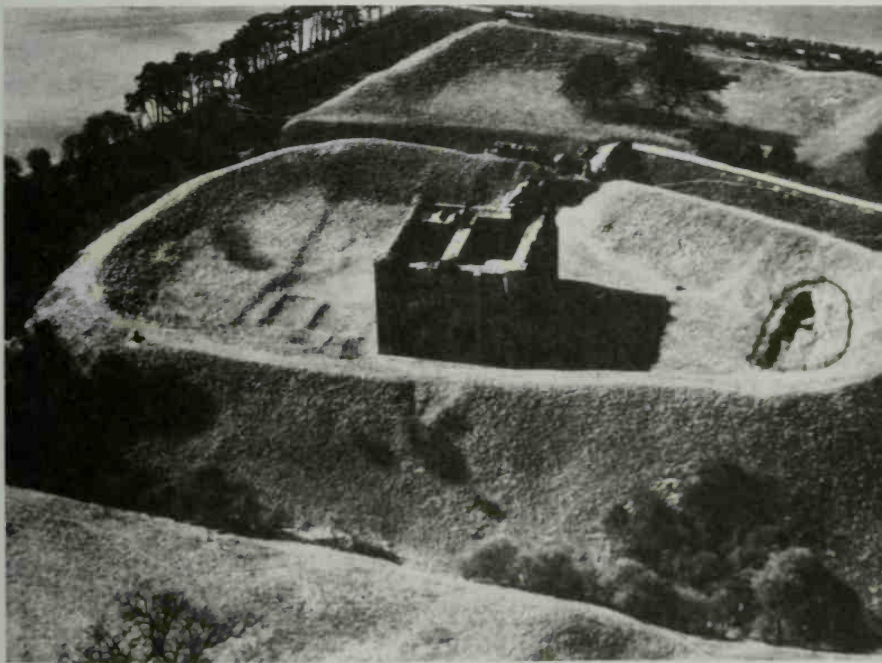
6 Castle Rising, Norfolk. The earthworks, which cover 13 acres, are probably pre-Norman. The keep is an excellent example of early Norman work. It measures 75 \times 64 ft and is 50 ft high
