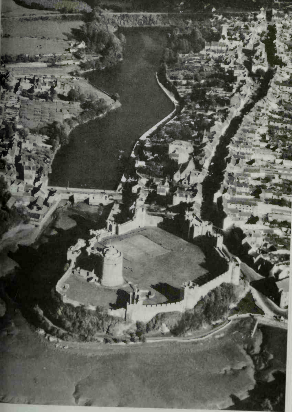
25 Pembroke. A castle guarding the mouth of a river. The keep was built in the late twelfth century and is 100 foot high; it has no buttresses, arcading or vaulting. It is roofed with a stone dome, and the walls are nineteen feet thick at the base. Similar – though not identical – keeps were built at Coucy and Bothwell
