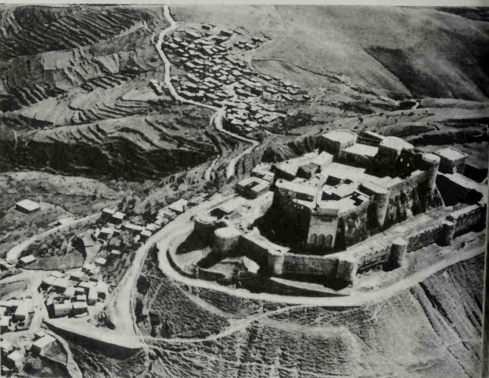
22 A view of Krak des Chevaliers, showing the concentric pattern and the flanking towers
