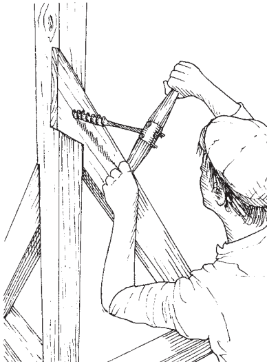
The dovetailed lap joint can also be fitted into an assembled frame, but is strong in tension as well as in compression.
