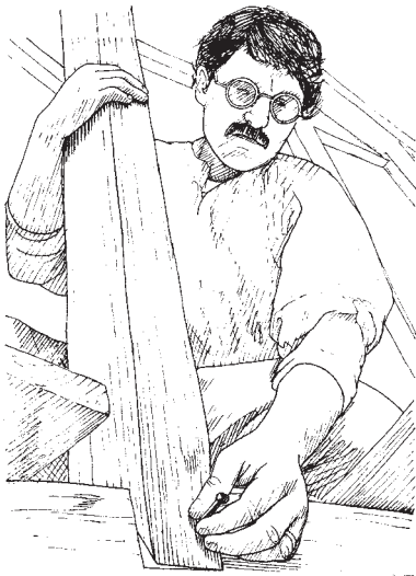
The miter lap joint allows you to fit a stud into an assembled frame.
