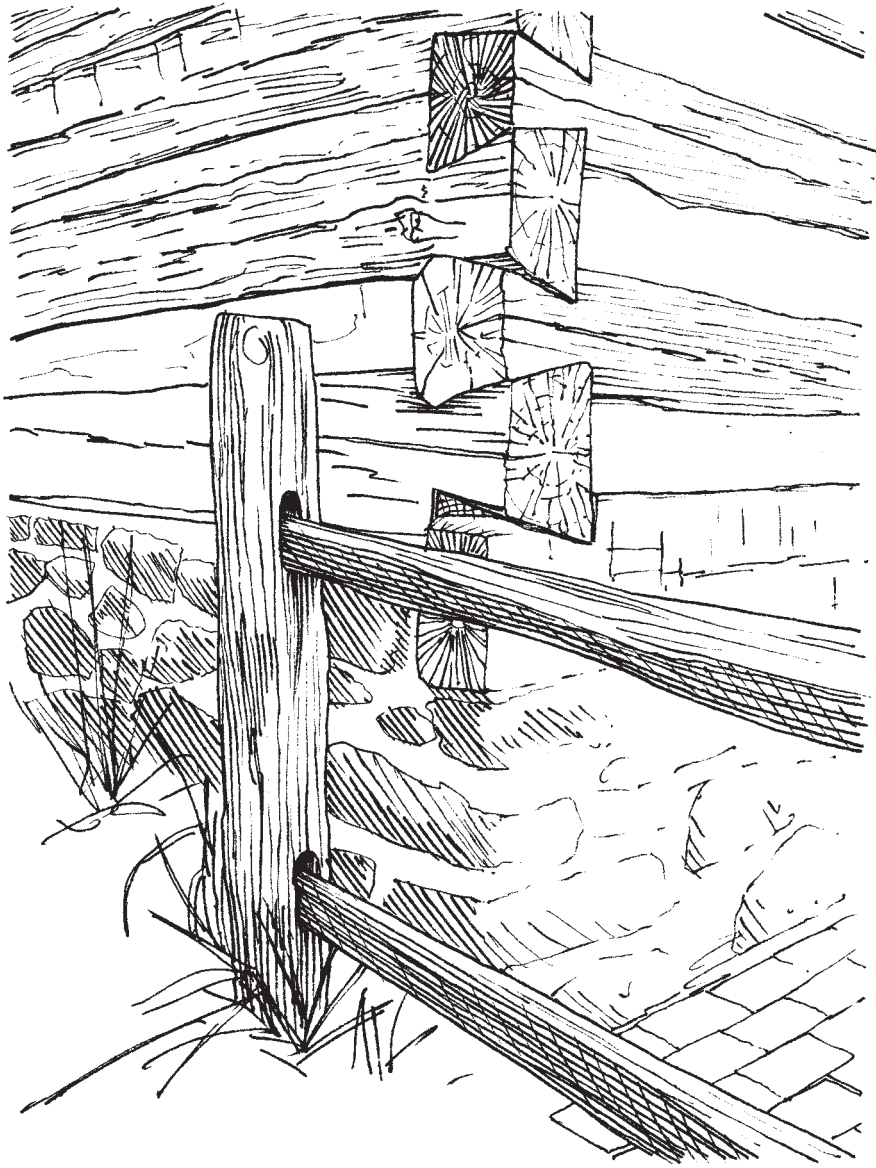
Full dovetails securely interlock the logs at the top and bottom yet still shed the rain.
