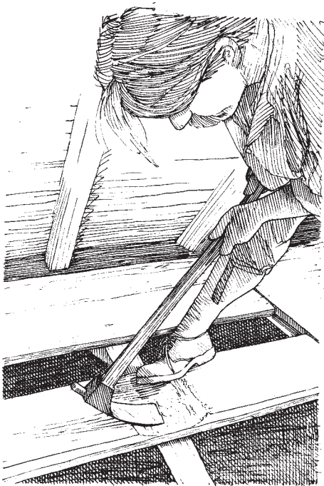
Adze floorboards to their lowest common thickness only where they cross a joist.
