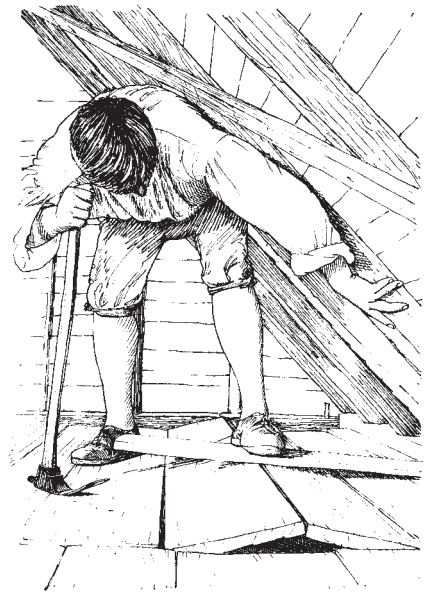
Nail boundary boards a bit too close together. This lets you spring the boards between them tightly into place.
