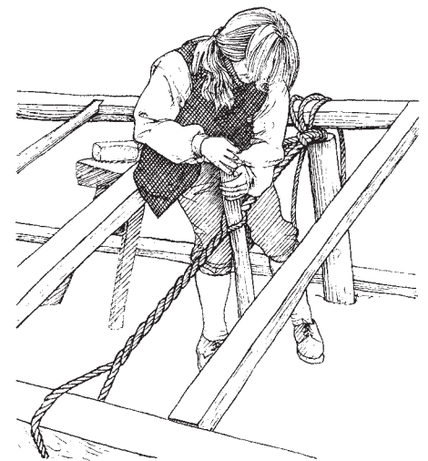
The Spanish windlass can help draw the frame together—and knock your teeth out if it slips.
