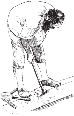
Cut the lower half of the lapped notch in the wall plate by sawing across the grain and then adzing out the waste.
