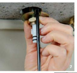
7. INSTALL THE SPOUT AND **SUPPLY.** Insert the spout in its hole, and slip the stopper rod through the back of the spout. Under the sink, put the washer and nut in place. The washer is slotted to fit around the stopper rod. Secure with an adjustable wrench or basin wrench. Don't overtighten—you could crack the sink. Connect the water-supply tubes to the faucet valves, and tighten with a wrench.
