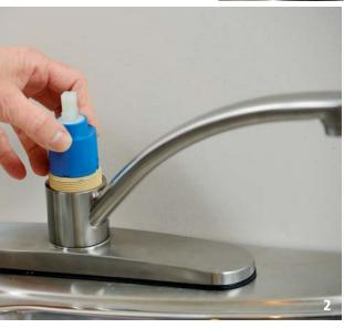
2. REASSEMBLE THE FAUCET. Put the cartridge back in place, and reinstall the clip if there is one. Screw on and hand-tighten the collar. Put the handle in place, tighten the setscrew, and pop the setscrew cap back into place.
