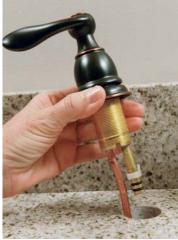
4. UNFASTEN THE VALVES. If there are setscrews securing the locknuts under the sink, loosen them. Then remove the locknuts and washers. Pull the valves out of the sink.
