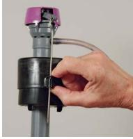
Newer toilets are designed to use less water than older models. If you want to save water with your older toilet, try moving the adjustment clip down an inch or two, adjusting until the flush is just powerful enough to do the job.
