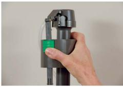
5. ATTACH THE REFILL TUBE. Slip the new refill tube onto the valve. If necessary, cut the refill tube to length. Clip or insert the tube into the overflow pipe. Turn on the water, flush, and make sure there are no leaks under the toilet. If there are, loosen the nuts securing the valve under the toilet, reseat the valve, and retighten the nuts.
