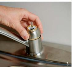
3. REMOVE THE COLLAR. Just grip the collar and unscrew it by hand.
