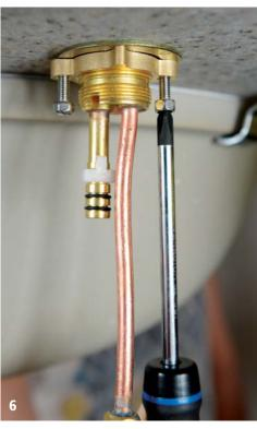
**6. INSTALL THE NEW VALVES.** Make sure the area around the sink holes is clean. If the sink top is uneven, put a bead of silicone on the gaskets under the faucet valves and the spout base. Put the valves and spout in place. Under the sink, secure the faucet valves with the washers and locknuts provided. If the nut has setscrews, tighten them.
