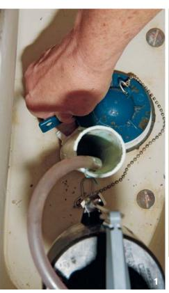
1. REMOVE THE FLUSH VALVE. Turn off the water supply to the toilet, and flush to empty the tank. Pull the flush valve off the pegs on the overflow pipe. Instead of attaching to pegs, some flush valves have a collar that fits over the pipe.
