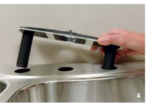
4. INSERT THE THREE-HOLE ADAPTER. The faucet shown can be installed in a one-hole sink and comes with an adapter for installation in a three-hole sink. Put the gasket under the adapter, and secure the adapter underneath with locknuts.
