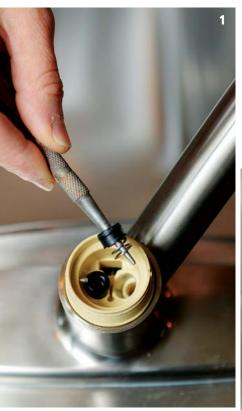
1. REMOVE THE SEATS AND SPRINGS. Once the ball is removed, use a nail set or similar tool to remove the two pairs of seats and springs. Replace them and any other parts that seem worn, especially any rubber parts that have become brittle.
