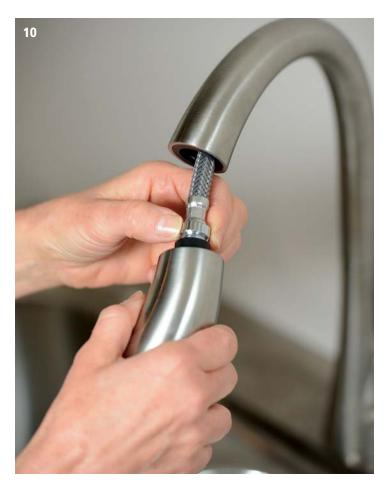
10. FLUSH THE LINES AND CHECK FOR LEAKS. Open the shut-off valves. Remove the sprayer head, and pull the hose into the sink. Turn the faucet handle to the mixed position, then flush the water lines for one minute. This will prevent any debris from getting into the sprayer head. Reinstall the sprayer head, and tighten the threaded connection as shown. Tighten any connections that leak.
