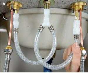
QUICK While you are tightening nuts under the sink, have a helper up top make sure the faucet valves and spout are centered over their holes and the handles are lined up correctly. If nobody is around, get everything snug and check topside before tightening.
