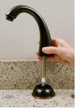
**5. REMOVE THE SPOUT.** Use an adjustable wrench or basin wrench to remove the nut securing the spout to the sink. Pull out the spout.
