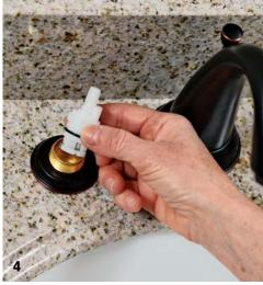
**4. PULL OUT THE CARTRIDGE.** This usually requires no tools. You might have to grab the cartridge with pliers and jiggle it a bit if it is stuck.
