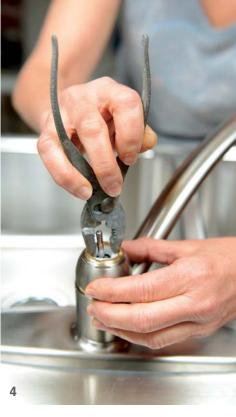
4. SCREW ON THE COLLAR. The ball may need to be pressed down against the springs so the cap tab can engage the notch to prevent the cap from rotating when you install the collar. With the tab aligned, put the collar in place. Use pliers to press down the cap while you start screwing on the collar.
