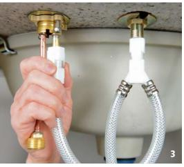
3. DISCONNECT THE MIXER TUBES. Double-handled faucets have tubes that bring the hot and cold water from the faucet valves to a junction fitting that sends water through the spout. Disconnect this tube from the faucet valves and spout using a wrench, if the connection fittings have nuts. This one has quick connects. Just pull out the tabs to release the connections.
