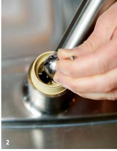
2. REASSEMBLE THE SEATS AND BALL. Install the new springs and seats, then insert the ball, aligning its slot with the pin in the faucet body.
