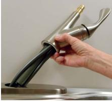
Faucets designed for three-hole-only installation don't have adapters—the hub is built into the escutcheon. These have no center nut, just two locknuts.
