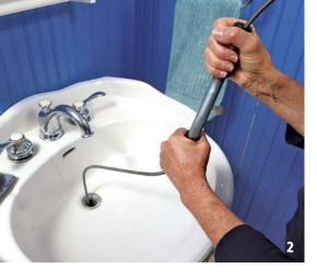
2. CLEAR THE DRAIN, Insert the boring head of the auger into the drain until you hit the clog. Slide the handle to a point near the sink and tighten the setscrew. Rotate the auger to clear the clog.
