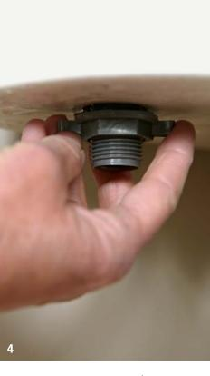
4. SECURE THE NEW VALVE. Under the toilet, hand-tighten the nut on the valve. Reconnect the water supply.
