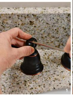
1. REMOVE THE CAP. Turn off the water at the supply valves under the sink as shown on p. 7, step 1, and open the faucet valves. Use a thin-blade screwdriver to pry the decorative cap off the faucet handle.
