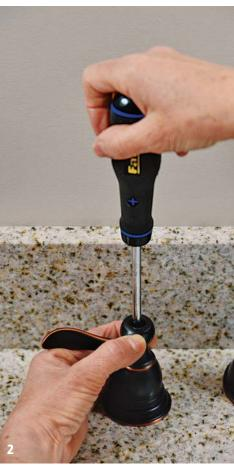
2. REMOVE THE HANDLE. Remove the screw that attaches the handle to the cartridge and take off the handle.
