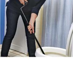
**USE A TOILET AUGER.** These augers are designed to navigate the serpentine trap built into toilets. Pull the cable up through the plastic sleeve, and insert the sleeve into the toilet. Then turn the handle to rotate the cable as you work it through the waterway. When you hit the obstruction, keep rotating to break it up.
