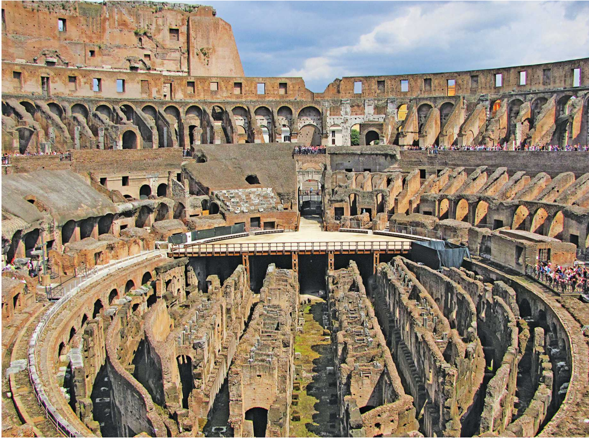
Figure 15.2. The interior of the Roman Colosseum, completed under Titus (emperor 79–81 CE). A floor was originally constructed over the maze of passageways now visible in the center, where gladiators, animals, and other entertainments were prepared prior to their entrance into the arena. The arena could even be flooded for the reenactment of naval battles. (Photo by author)
