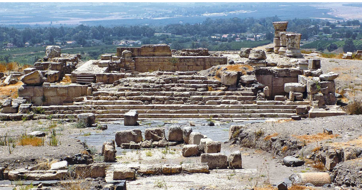
Figure 6.6. The foundations of an imperial cult temple a few miles south of Caesarea Philippi, itself a city full of pagan shrines in a largely Gentile area. This may have been one of three such temples to Augustus and Roma, the other two having been identified at Caesarea Maritima and Sebastia (formerly the city of Samaria). (Photo by author)
