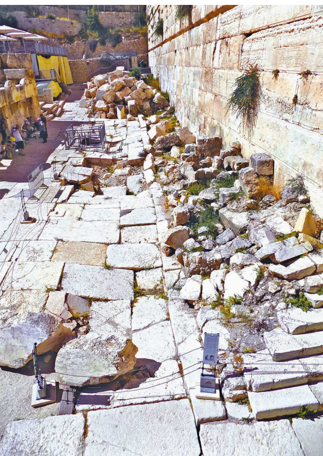
Figure 7.1. The first-century street alongside the southwest corner of the Temple Mount shows the damage caused as Roman legionaries (and, no doubt, Jewish captives) threw down the stones constituting the fortified walls surrounding the temple courts following their victory in 70 CE. Many of the large ashlars remain piled where the Romans threw them at the head of the excavated street. (Photo by author)
