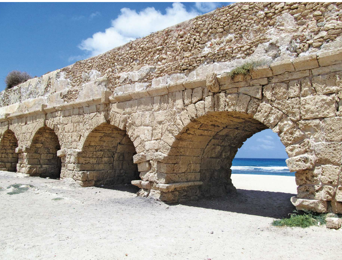
Figure 16.3. A section of the double aqueduct carrying water to Caesarea Maritima from a source seven miles to the north. The first aqueduct was ordered built by Herod the Great in connection with his refounding of the city; the second was built under Hadrian to meet the city's growing needs. Some scholars speculate that Paul wrote Philippians during his two-year detention in Caesarea. (Photo by author)
