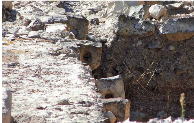
Figure 6.7. Mooring stones built into the harbor seawall at Magdala (Taricheae), a major hub of the fishing industry in the Sea of Galilee known especially for preparing fish for export. Fishermen from other towns might well have sought to sell their hauls to the preparers here. (Photo by author)
