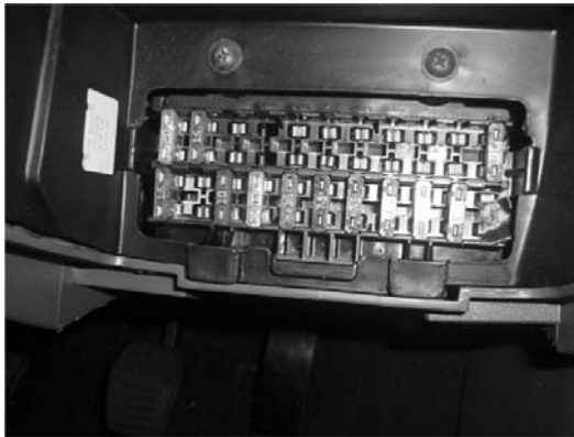
Figure 3.138 CJB, relays are behind the fuse box
