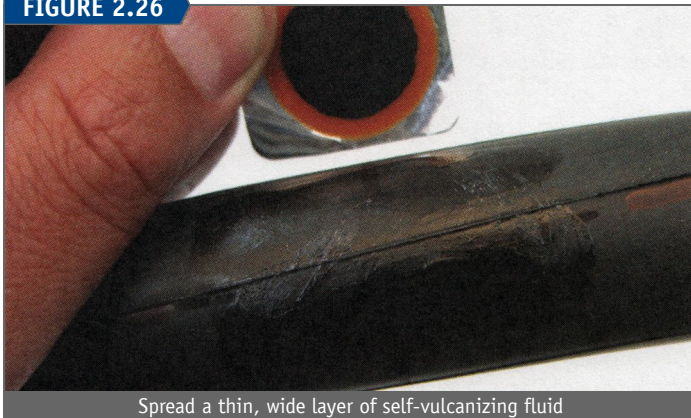
Spread a thin, wide layer of self-vulcanizing fluid
