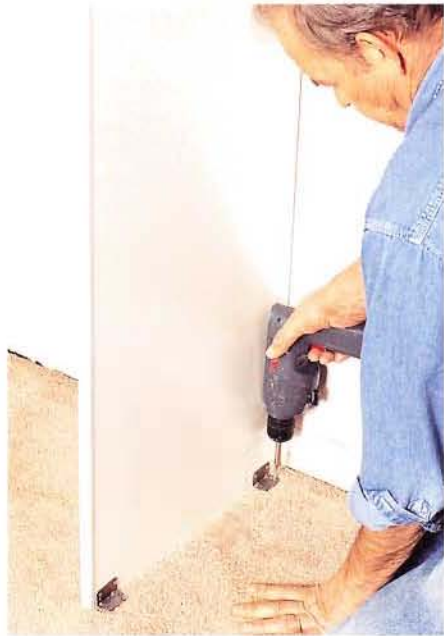
Hang wall cabinets in your closet work space using 3" screws driven into the studs. The two side walls and back wall allow us to install all types of cabinets and bookcase storage units.
