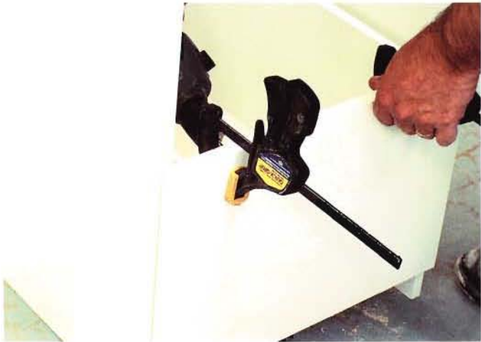
Cabinet doors and drawer faces are low-cost alternatives for the closet work center cabinets. Cut the boards to size, tape the edges and install.
