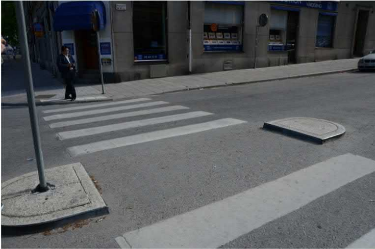
FIGURE 2.11 A safe island in the middle of the street to provide a safe space for pedestrians crossing the street.
