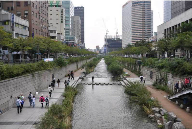
FIGURE 7.23 Hydrophilic platform in the middle section of Cheonggyecheon with stone and plant revetment.
