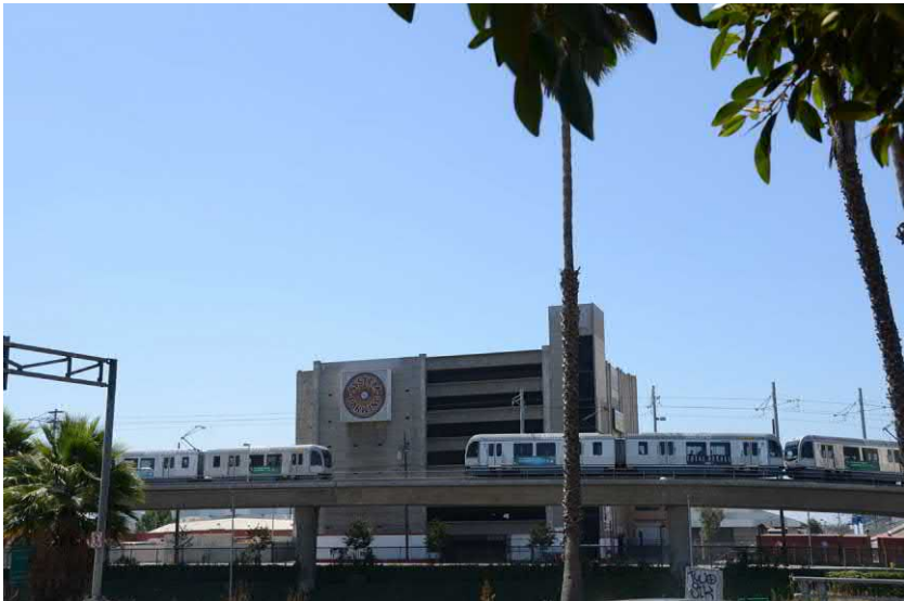
FIGURE 20.3 Elevated light rail in downtown Los Angeles.
