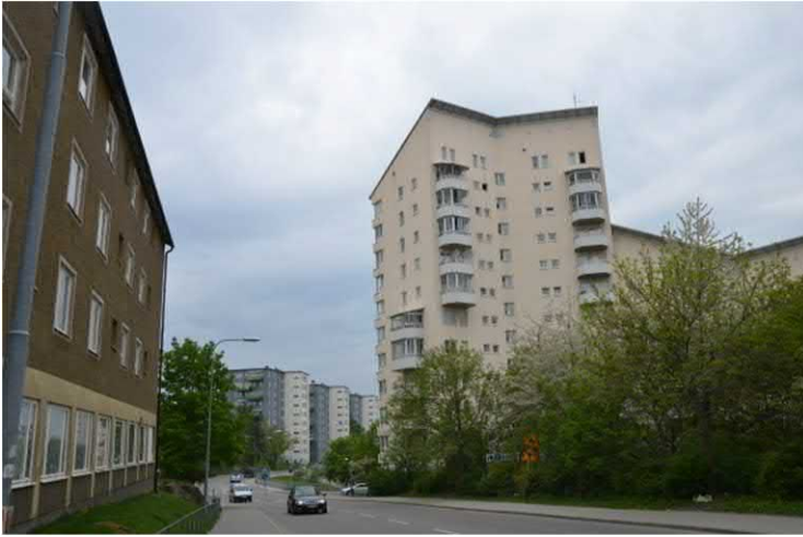
FIGURE 2.16 High-rise residential apartment in Vällingby community.
