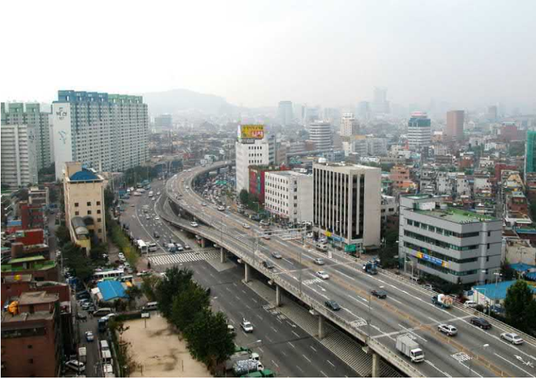
FIGURE 7.20 Before the restoration project, a highway on the river, with the river was underneath.
