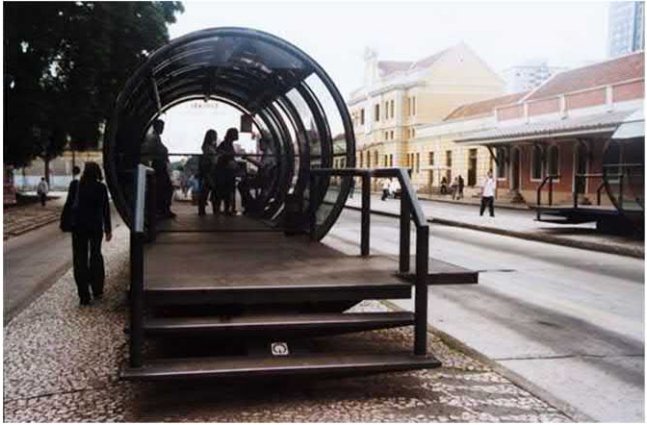
FIGURE 4.5 The inside of a tubular station.
