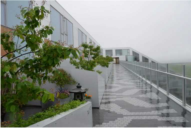
FIGURE 1.14 Open-air gardens in front of each entrance, which is directly connected with the outer corridor.
