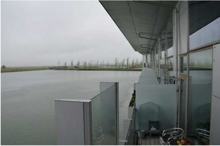
FIGURE 1.15 Waterfront housing with a rainwater lake.
