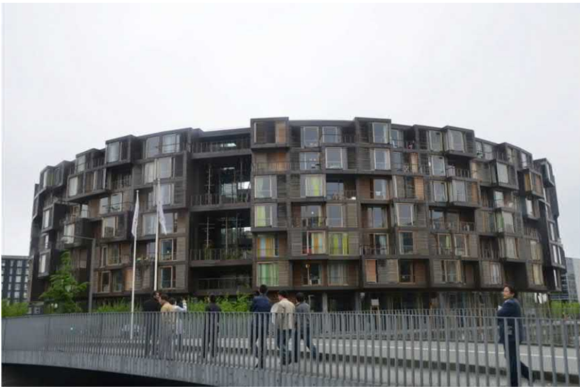
FIGURE 1.20 The circular dormitory building of the University of Copenhagen.
