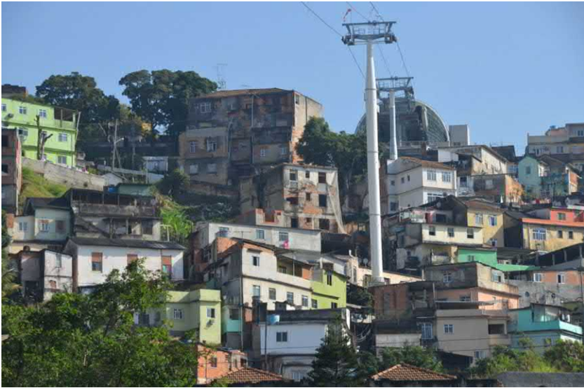
FIGURE 15.12 Construction of a cable car to a hilltop slum.
