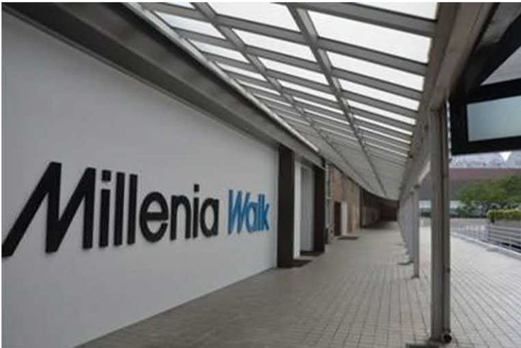
FIGURE 3.15 The corridor of the building itself.
