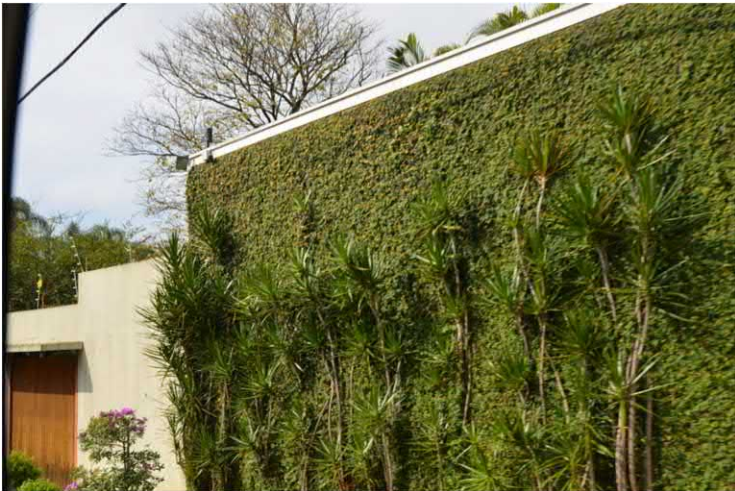
FIGURE 19.6 Vertical greening of walls fills buildings with vitality.
