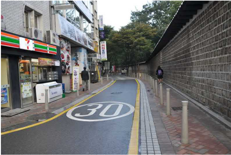
FIGURE 7.8 Guardrails to separate pedestrians from motor vehicles.
