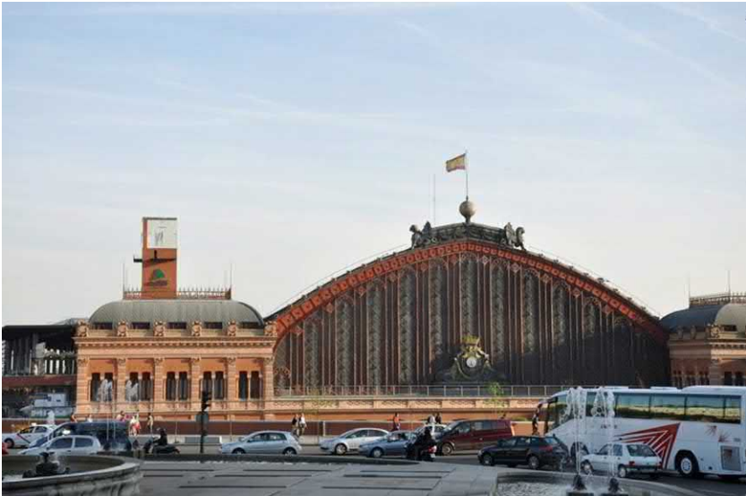
FIGURE 12.14 Old building of Atocha railway station.
