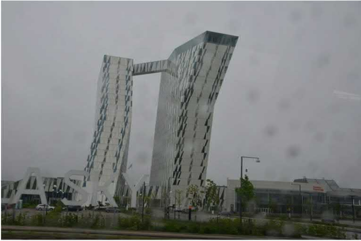
FIGURE 1.22 Architectural shape of the Bella Sky Hotel.
