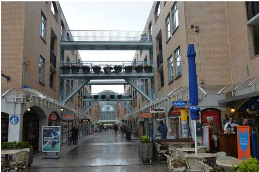
FIGURE 10.20 Residential buildings are built on the upper floors of commercial shops, and interconnected by air corridors.
