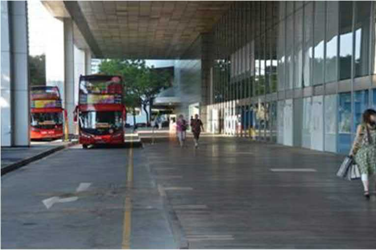
FIGURE 3.16 A broad sunshade roof above a bus station connected to a building.
