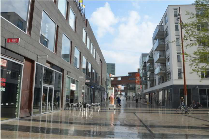
FIGURE 10.21 Residential buildings above commercial shops.
