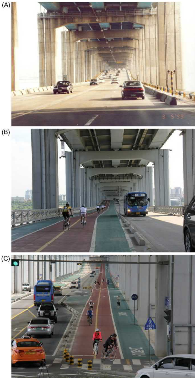
FIGURE 7.5 The changes to Diving Bridge passing over the Han River (1999–2013). (A) Two-way four-lane road solely for motor vehicles in 1999; (B) half of the road was converted into a bicycle and pedestrian way in 2013; (C) the south entrance of the bridge in 2013.
