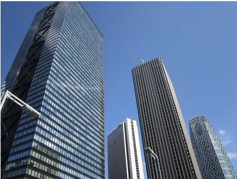
FIGURE 5.11 High-rise buildings that can be reached by walking from Shinjuku station via the underground passage in about 5 min.
