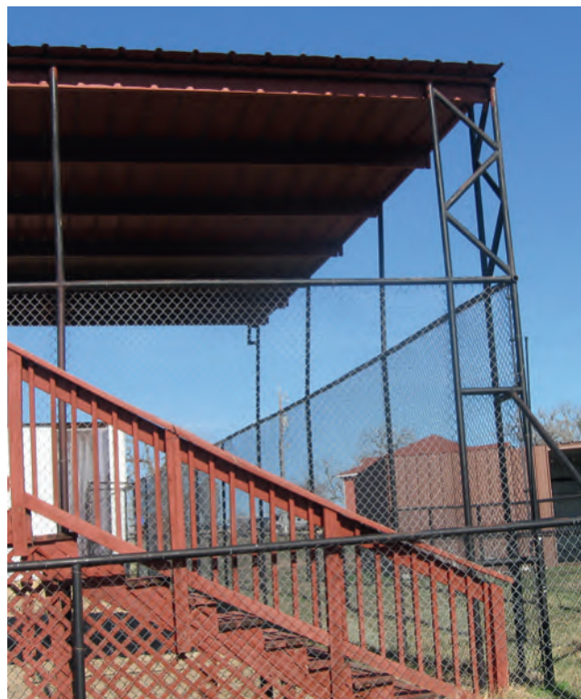
• Figure 87.1 Giraffe ( Giraffa sp.) shade structure with openings large enough for the head or ossicone; may cause a fatal entrapment.
