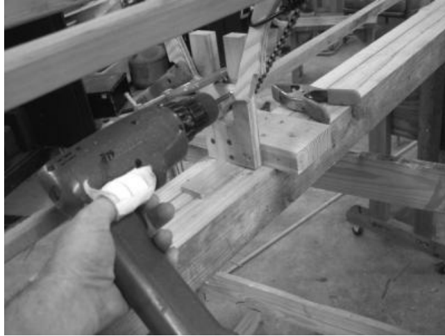
Driving screws through the frame
