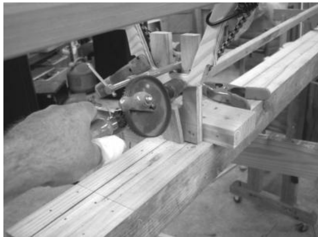
Drilling pilot holes
