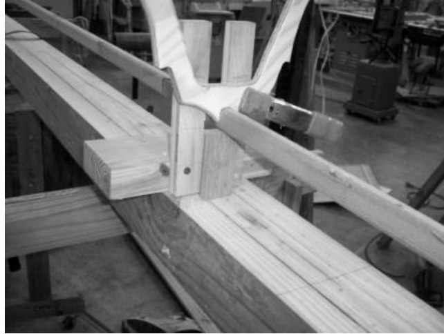
Frame temporarily clamped to the bracket
