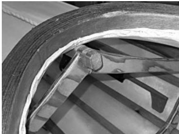
Single deck beam
