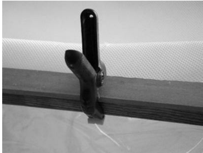
Batten clamped in place
