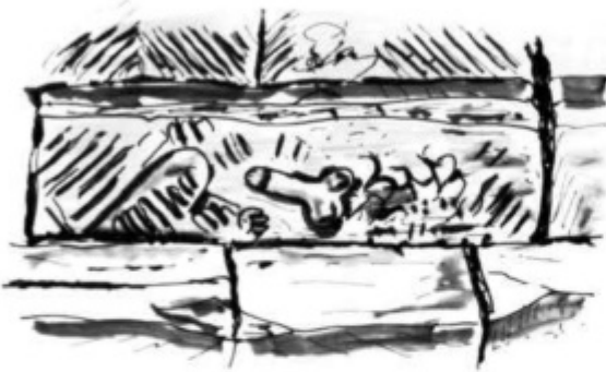
Fig. 66b Phallus on the bridge abutment at Chesters.
