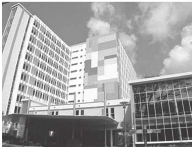
FIGURE 5.3.2.0.1 Picture of the buildings.
