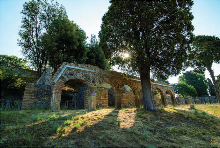
Figure 2.5 Colonnaded shops at Pompeii's Porta Ercolano suburb. (Photo: author, courtesy of the Ministry for Cultural Heritage and Environment. Reproduction or duplication by any means is forbidden.)
